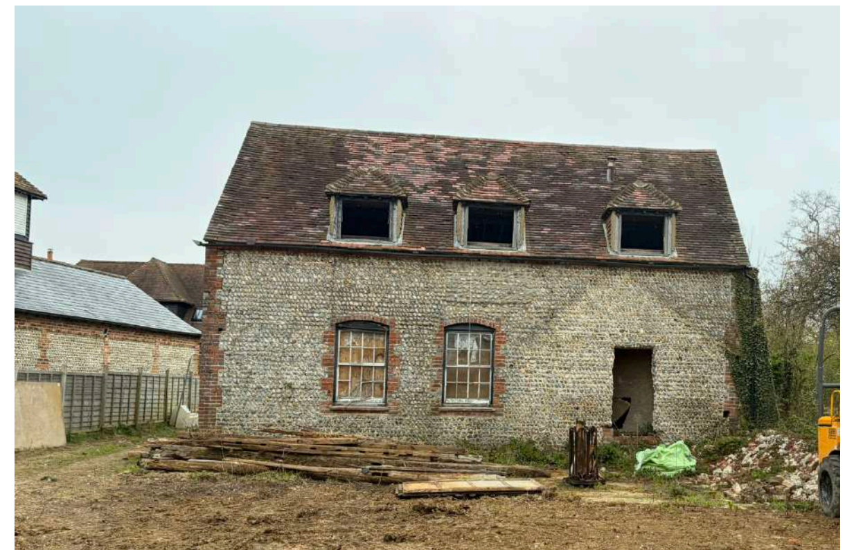
South elevation of Forest Barn; the ghost of the recently lost south extension is seen in the flintwork
