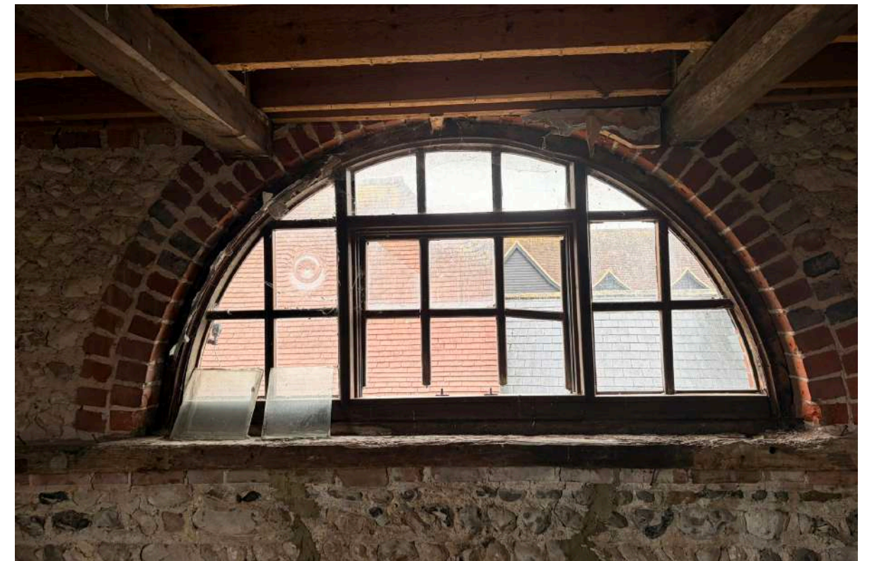
Interior of west elevation; the historic form and fabric is evident, with the later inserted timbers of the first floor above having interrupted the interior space
