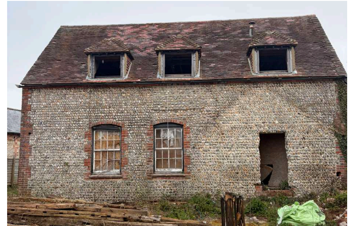
South elevation of Forest Barn, 2026
