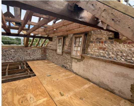
Plate 5: Eastern Roof Void
