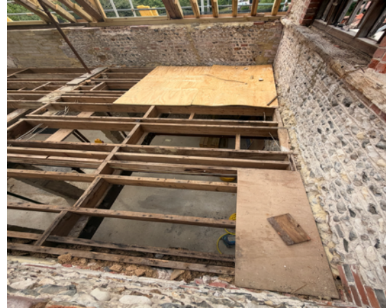
Plate 8: Western Roof Void
