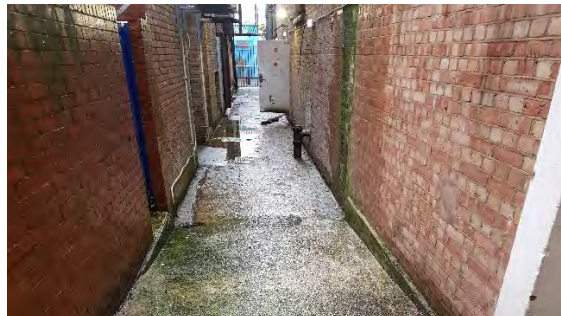
Photo 10. Looking east towards Bath Place – Northern drainage route via passage to rear of Marine Parade.
