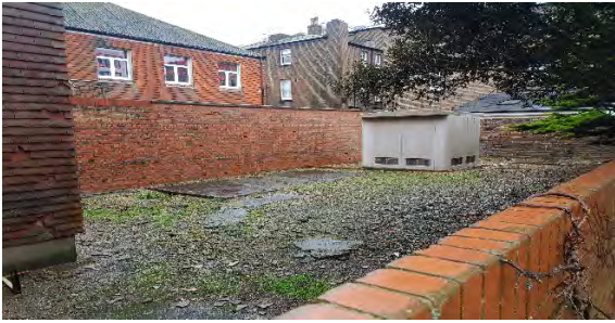
Photo 1. Location of proposed extension looking towards existing Sub-station.
