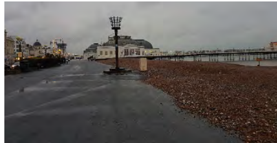
Photo 6. Looking east along esplanade towards the pier.
