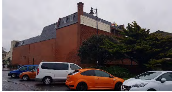
Photo 2. Looking towards site from Montague Place.
