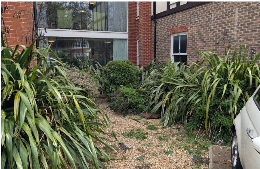
Photo 12 – Introduced shrubs requiring removal to enable the extension.
