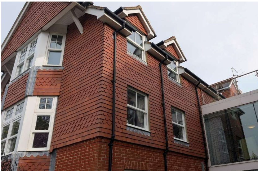
Photo 3 – South corner of north wing, where hanging tiles would require removal.
