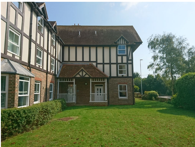
Figure E- existing gardens located on Wykeham Road and view towards the existing unused ground floor verandah
