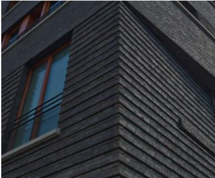
7 - Dark grey brick to the base of the block
