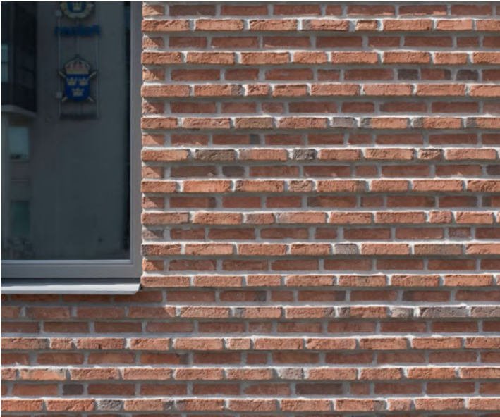
5 - Protruding brick detailing adjacent to windows
