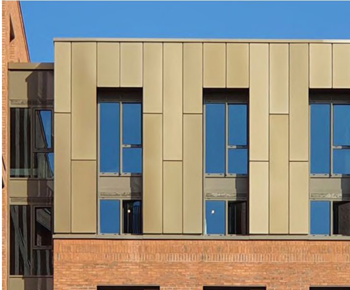
1 - Penhouse cladding in a non-reflecting light brass colour
