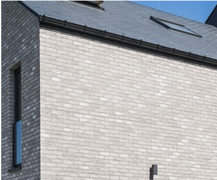
4 - Light grey facing brick to the upper levels
