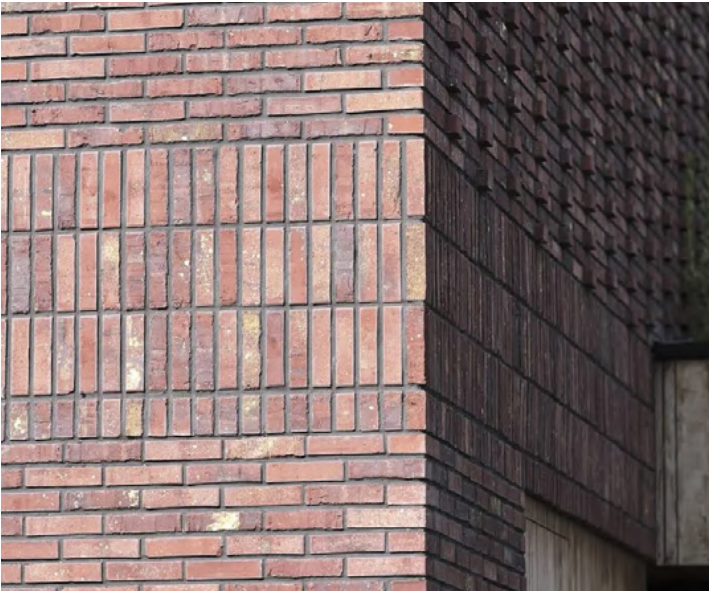
8 - Vertical brick soldier course banding detail between floors
