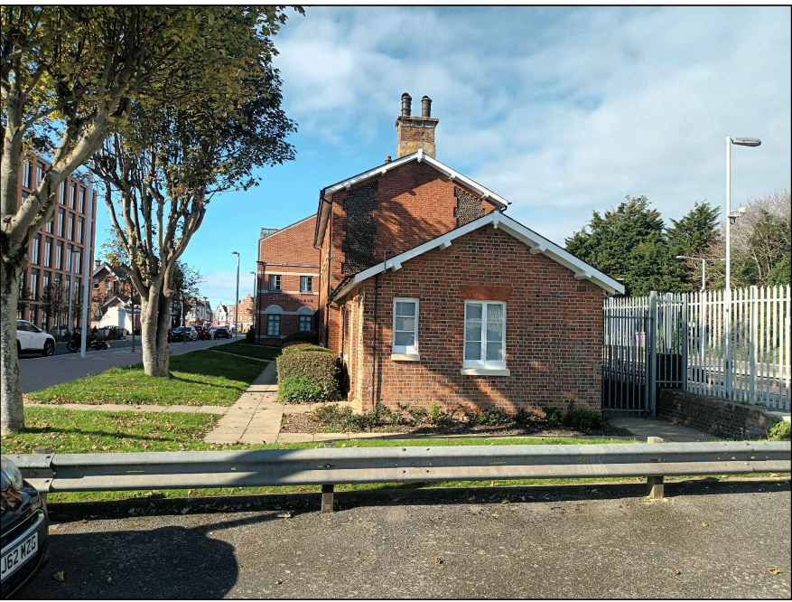
East Wing Side
