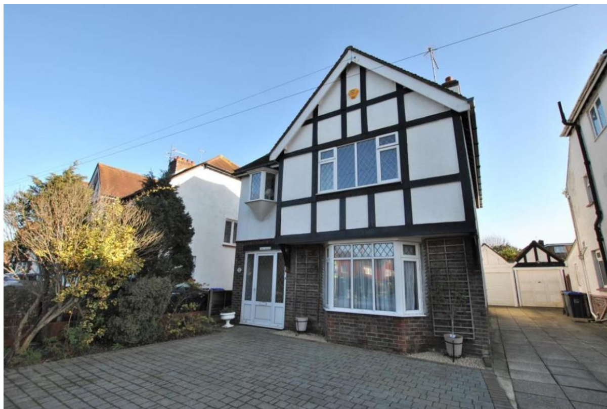
Fig 1 Front elevation of 60 Southwick Street
