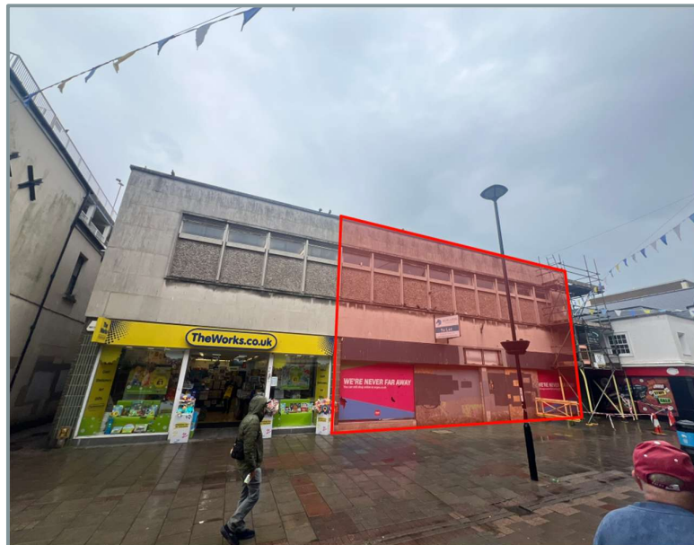
The site (shaded red) and adjacent building
