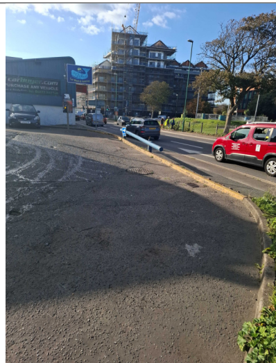
Other Site Photos: FOUL MH ON CAR WASH PROPERTY
