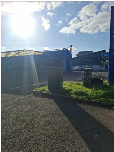
Other Site Photos: PUMP STATION PANEL
