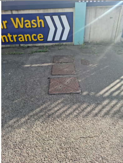
Other Site Photos: 3 STAGE IC
