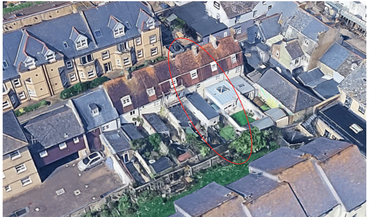
Aerial image showing the pattern of rear extensions to 16-26 West St.
