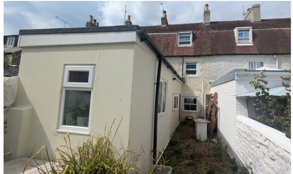
Existing kitchen-utility extension seen from the rear, with UPVC fascia, felt roof and UPVC windows. Even at midday in the height of summer the side passage is shaded.
