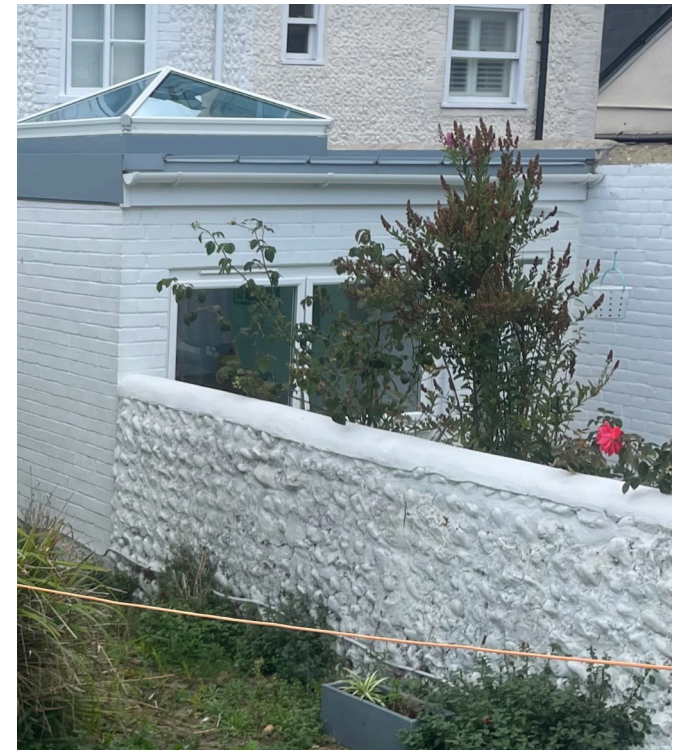
Neighbouring extension with painted brickwork, standing seam roof and aluminium window. The proposed rooflight to 22 West St would be less prominent, and the roof colour would be darker.
