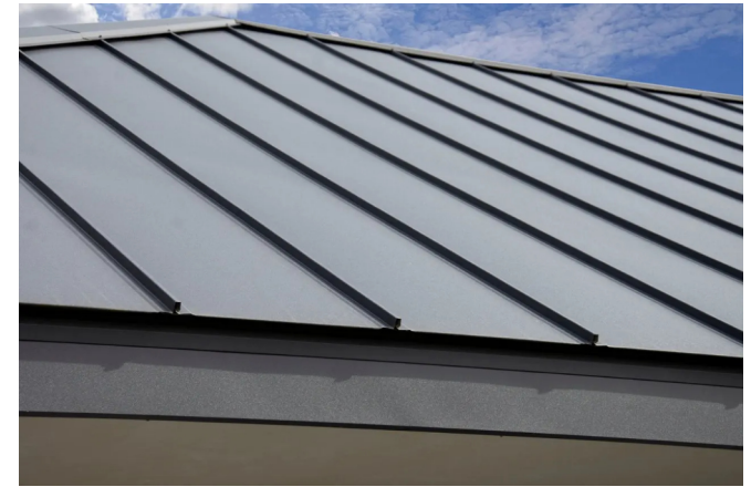
Example standing seam roof in lead-grey colour.
