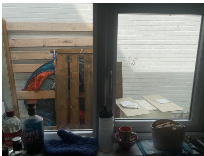
Existing kitchen window facing north and looking onto a blank wall.
