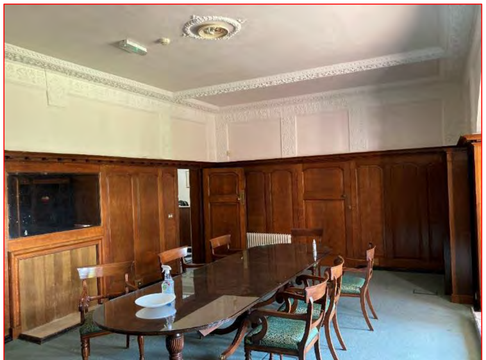
Plate 20 View of eastern end of Room GF4. Note that the timber panelling dates from the early 20 th century. Note this image is from 2021 prior to the building's renovation, though all historic fixtures, fittings and finishes have been retained.
