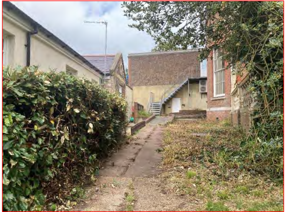
Plate 8 Part view of largely blind south elevation to the two-storey westernmost wing (centre). Note that the buildings in left of picture do not form part of the site. Note this image is from 2021 prior to the building's renovation.
