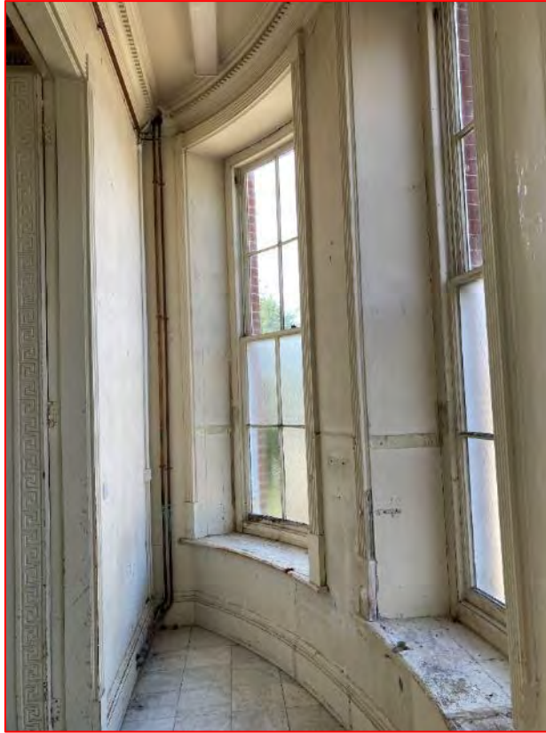
Plate 24 Partial view of curved bay at western end of Room GF5. Note this image is from 2021 prior to the building's renovation, though all historic fixtures, fittings and finishes have been retained and restored to a high standard.
