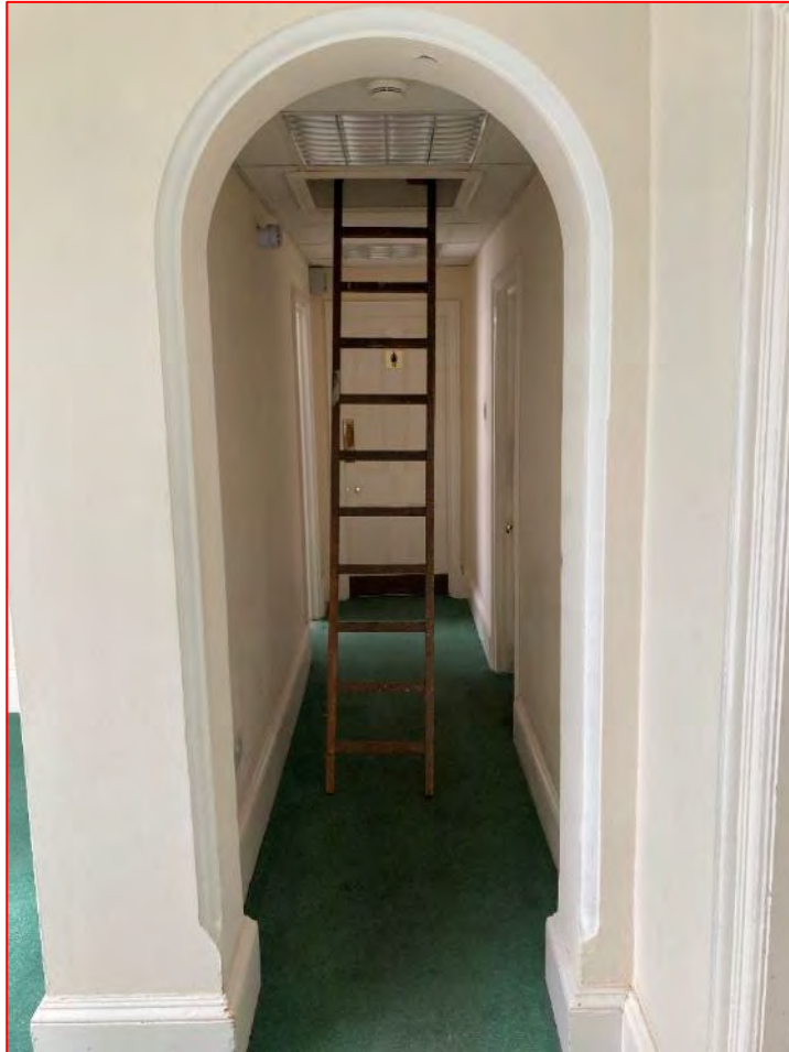
Plate 43 View of corridor leading to existing toilets at second floor level. Note this image is from 2021 prior to the building's renovation, though all historic fixtures, fittings and finishes have been retained and restored to a high standard.
