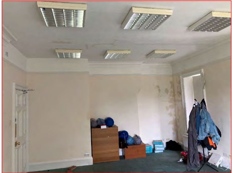
Plate 32 View of western end of Room FF1 (2021) illustrating the lack of any historic fixtures and fittings. Note this image is from 2021 prior to the building's renovation, though all historic fixtures, fittings and finishes have been retained and restored to a high standard.
