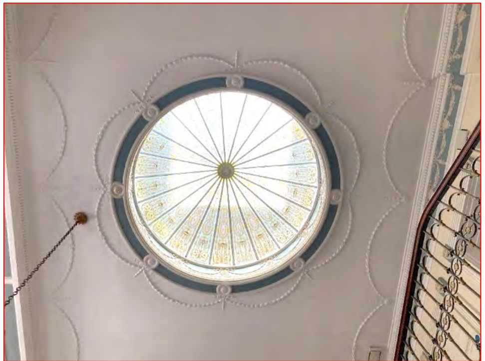
Plate 12 Adam style dome located above main entrance stair. Note this image is from 2021 prior to the building's renovation, though all historic fixtures, fittings and finishes have been retained.
