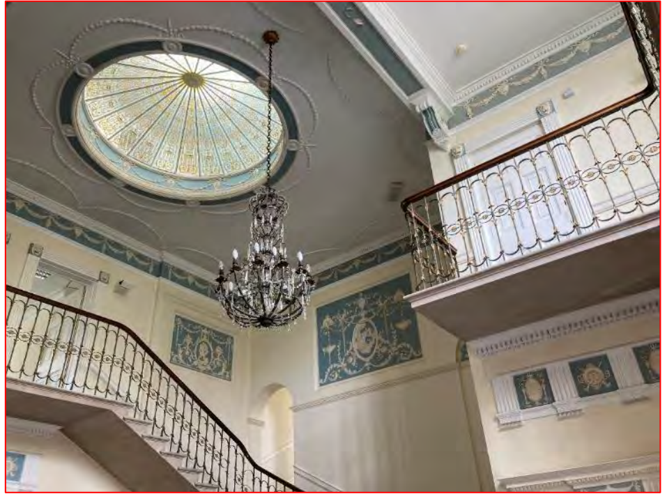
Plate 11 Part view of ceiling above main ground floor staircase. Note that this elevation was remodelled in the early 20th century. Note this image is from 2021 prior to the building's renovation, though all historic fixtures, fittings and finishes have been retained.
