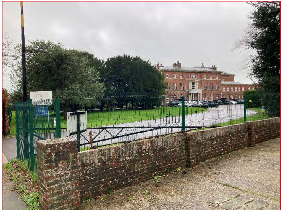
Plate 1 Principal north elevation to the Courtlands building taken from Parklands Avenue looking south-west. Note that this elevation was remodelled in the early 20 th century.
