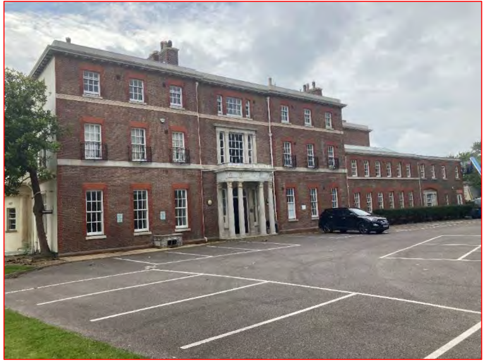
Plate 2 Principal north elevation to the former Courtlands Hospital building, taken from the lawned area to the north-east. Note the three-storey element, which is earlier in date with the two-storey element having been added at a later date. Note this image is from 2021 prior to the building's renovation.
