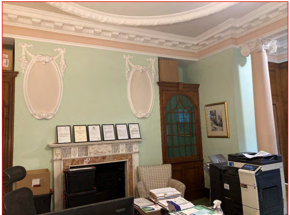
Plate 18 View of eastern part of Room GF3 showing the Adam style plasterwork and fire surround. Note the column (in right of picture).
