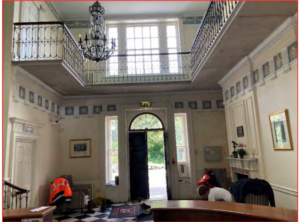
Plate 9 View of main entrance hall and door at ground level. Note this image is from 2021 prior to the building's renovation, though all historic fixtures, fittings and finishes have been retained.
