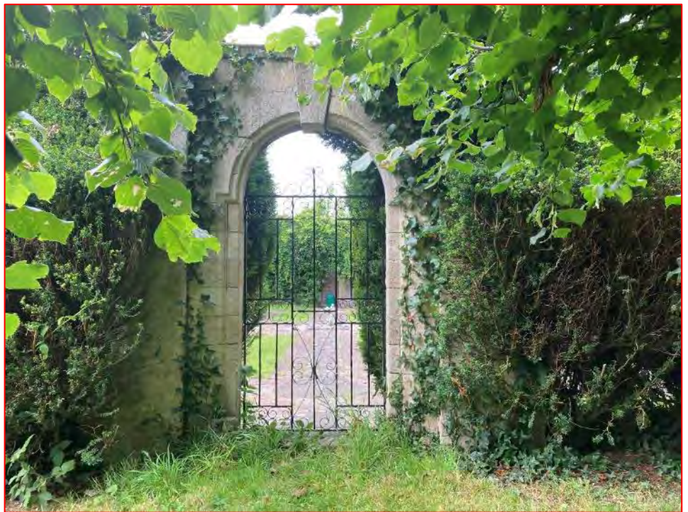
Plate 47 View of the listed stone archway located in the garden area to the south of the Courtlands building.
