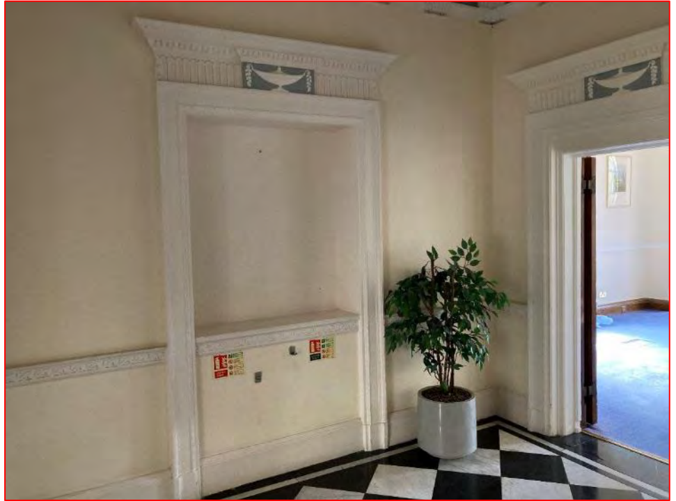
Plate 13 View of the infilled door opening to the secondary stairwell at the eastern end of the building. Note the door opening to the south-east room is evident (right of picture). Note this image is from 2021 prior to the building's renovation, though all historic fixtures, fittings and finishes have been retained.
