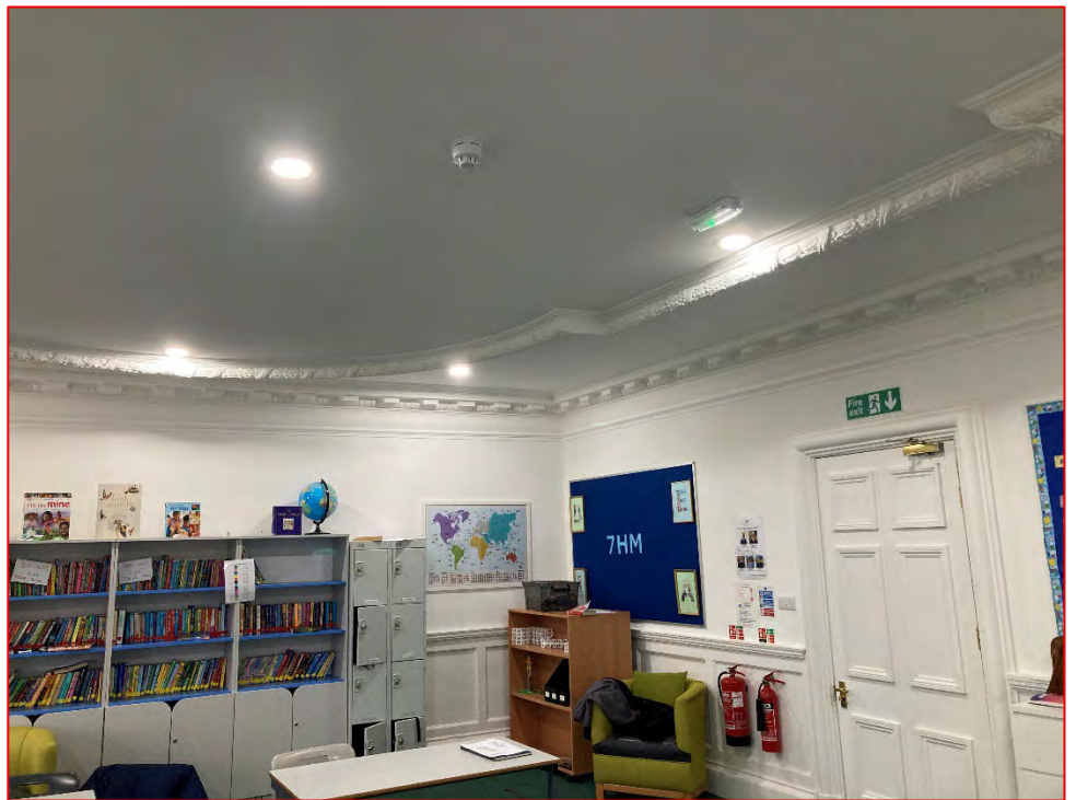
Plate 36a Room FF4 following its renovation as part of the conversion of the building into a school illustrating the high standard of decorative finish that is evident throughout the building.
