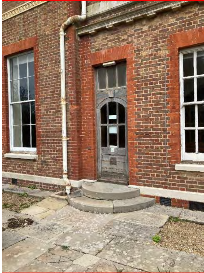
Plate 5 Example of ground floor door opening to the south elevation of the Courtlands building. Note this image is from 2021 prior to the building's renovation.
