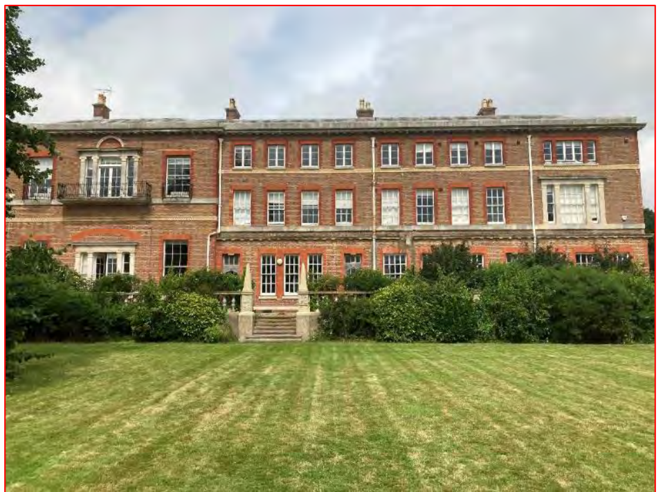
Plate 4 View of south (garden) elevation to the Courtlands building. Note this image is from 2021 prior to the building's renovation.
