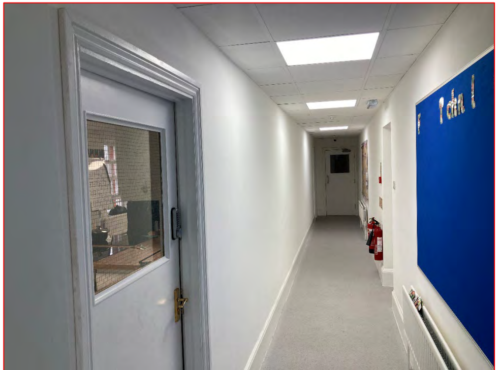
Plate 28a Image showing one of few new partition walls within the building (left of image). The teaching space through the door on the left is used for food technology and as part of fire compartmentalisation, this stud partition was inserted creating a corridor.
