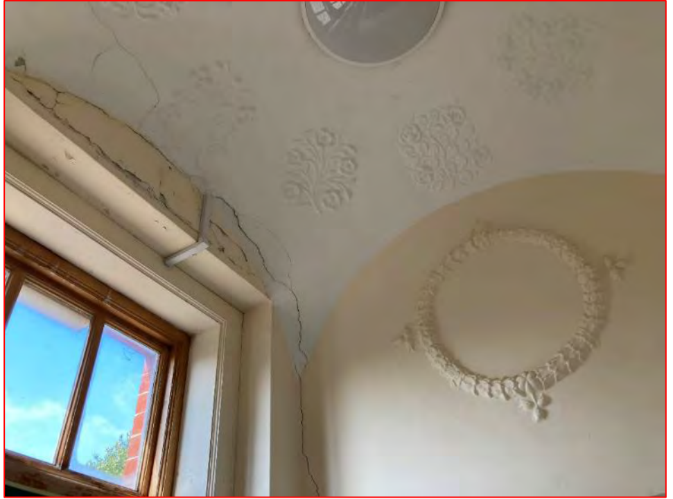
Plate 17 High level plasterwork located within the lobby between rooms GF2 and GF3. Note this image is from 2021 prior to the building's renovation, though all historic fixtures, fittings and finishes have been retained.
