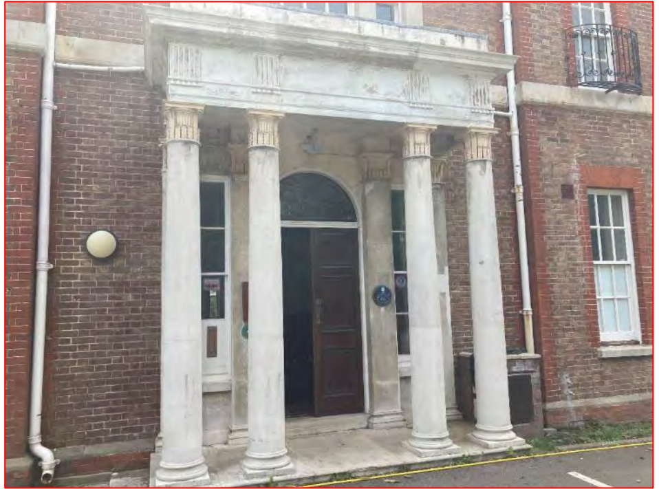
Plate 3 Main entrance porch to the north elevation. Note this image is from 2021 prior to the building's renovation.
