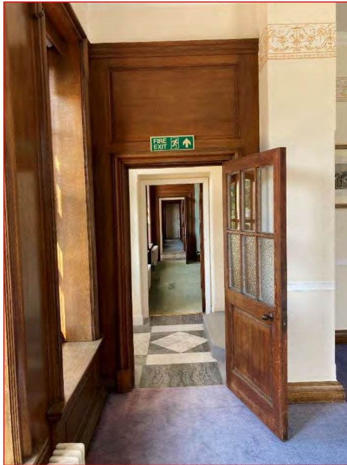
Plate 16 View of door to lobby between rooms GF2 and GF3. Note that this view is taken from Room GF2. Note this image is from 2021 prior to the building's renovation, though all historic fixtures, fittings and finishes have been retained.
