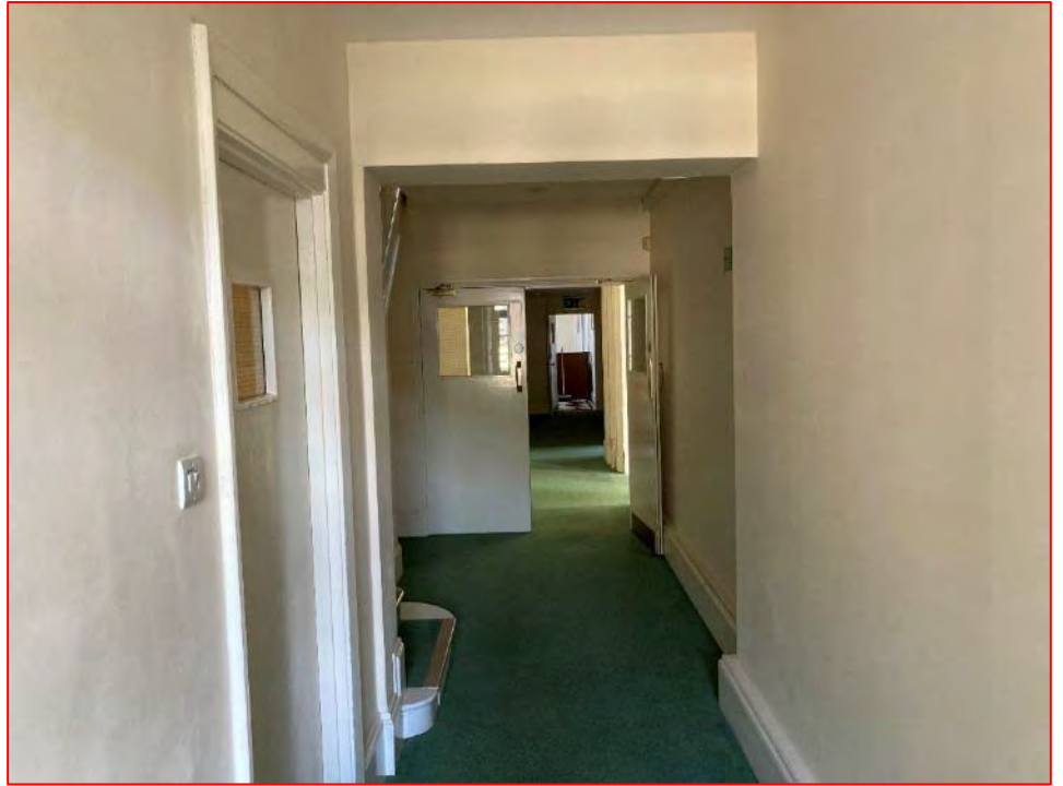
Plate 25 View of corridor to immediate north of Room GF5. Note that this view looks east towards the main entrance hall. Note this image is from 2021 prior to the building's renovation, though all historic fixtures, fittings and finishes have been retained and restored to a high standard.
