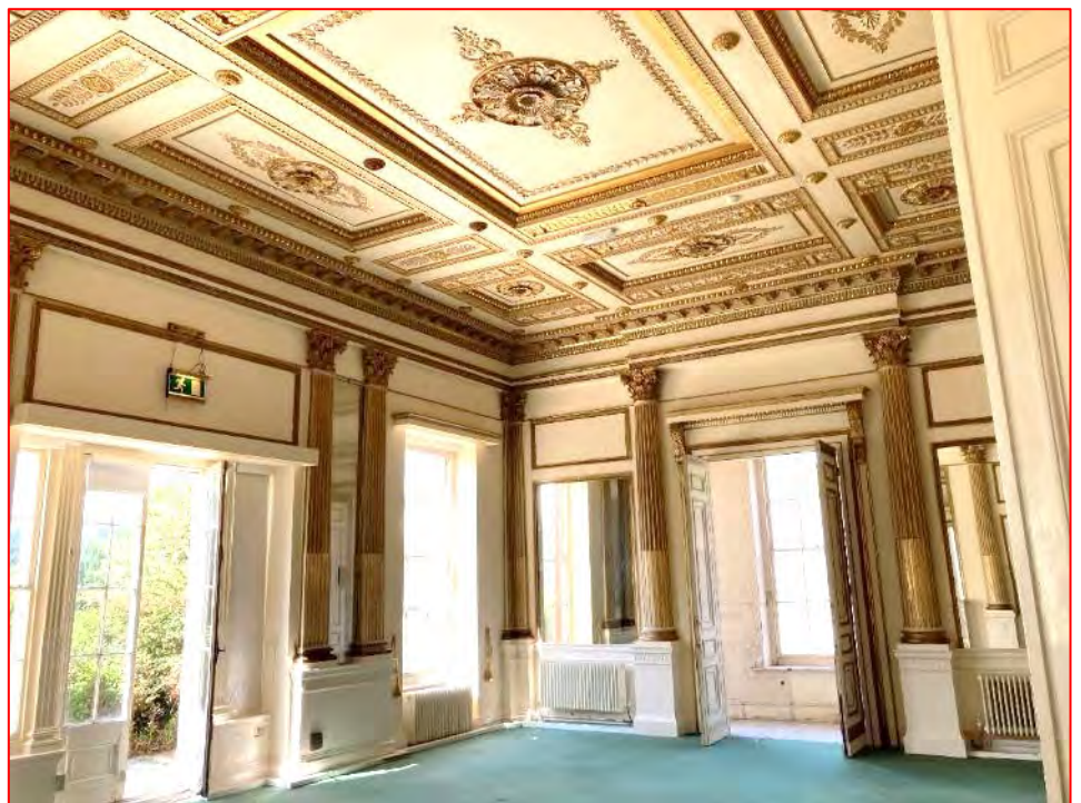
Plate 22 Part view of southern and western end of Room GF5 (historic Drawing Room). Note this image is from 2021 prior to the building's renovation, though all historic fixtures, fittings and finishes have been retained.
