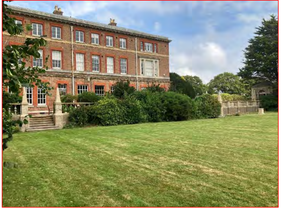
Plate 44 View of listed terrace taken from the garden area to the south.
