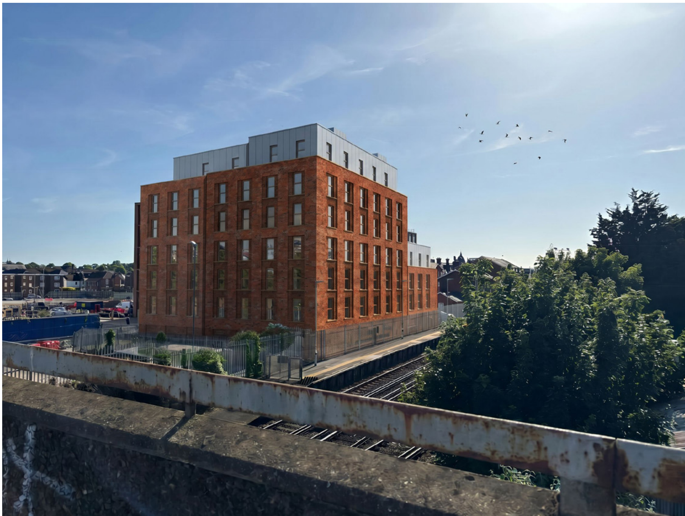
Visual 3 : View from Broadwater Road Bridge looking southwest (Sent to Louise Prew for comment on 4th June 2026).
