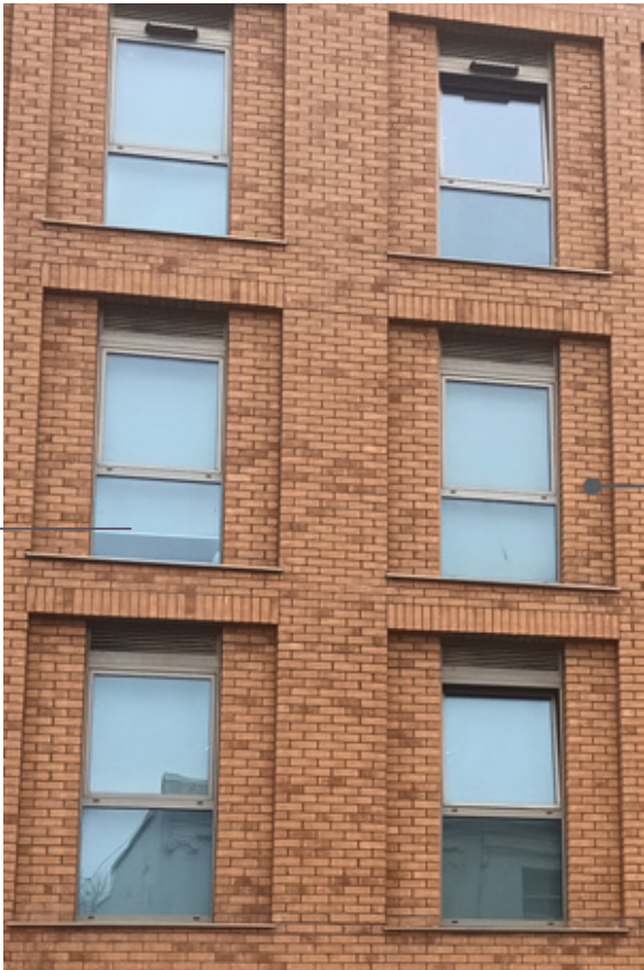
Fenestration set within recessed brickwork panels
