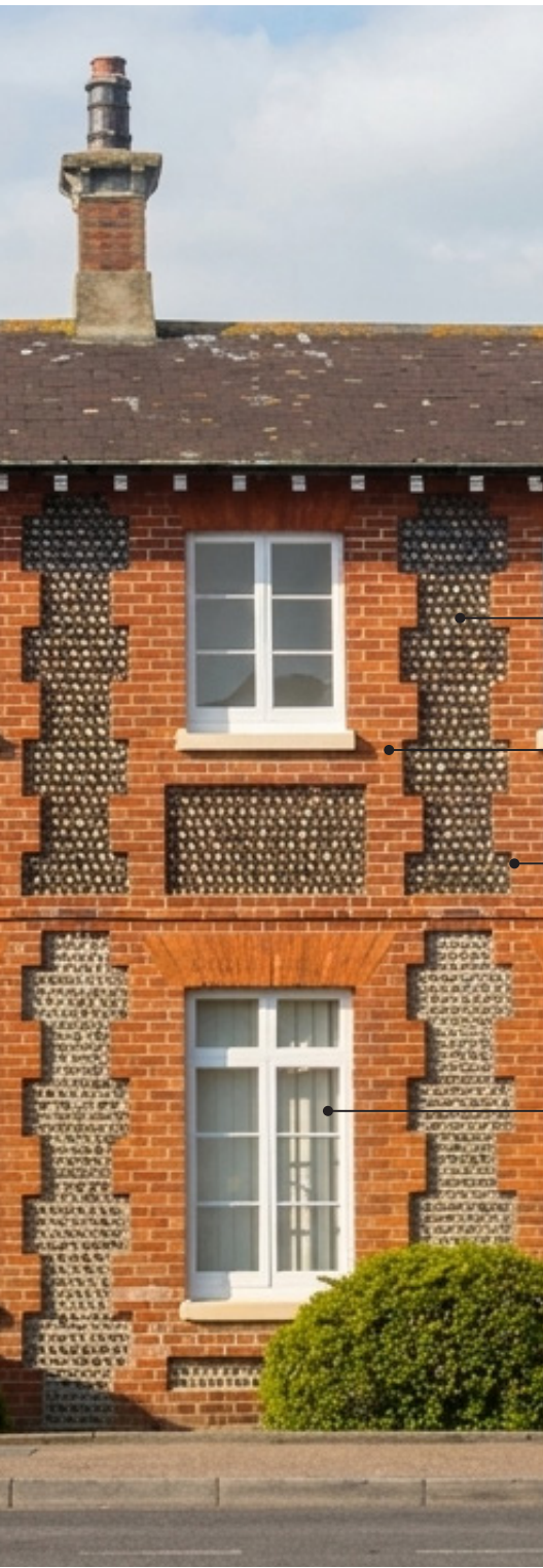
Existing Heritage Building Detail Showing Fenestration Hierarchy and Material Palette.
