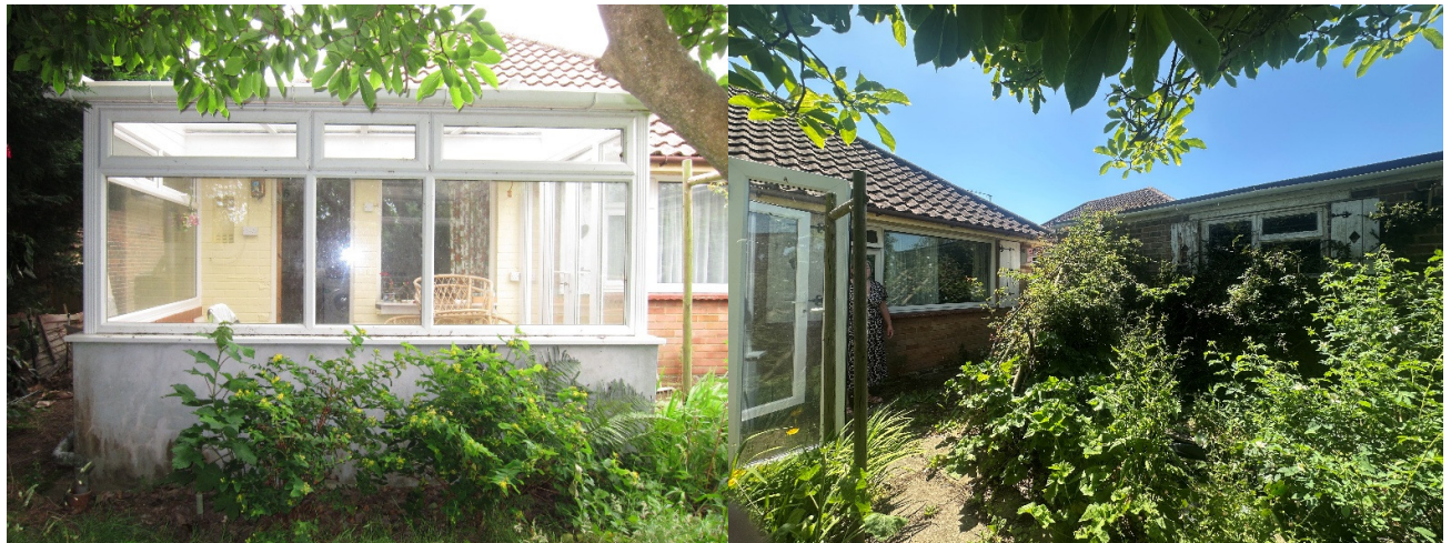
Rear of house
