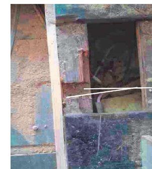
Existing notch in joist 1
