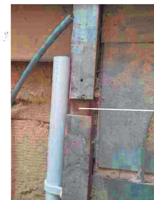
Existing notch in joist 2
