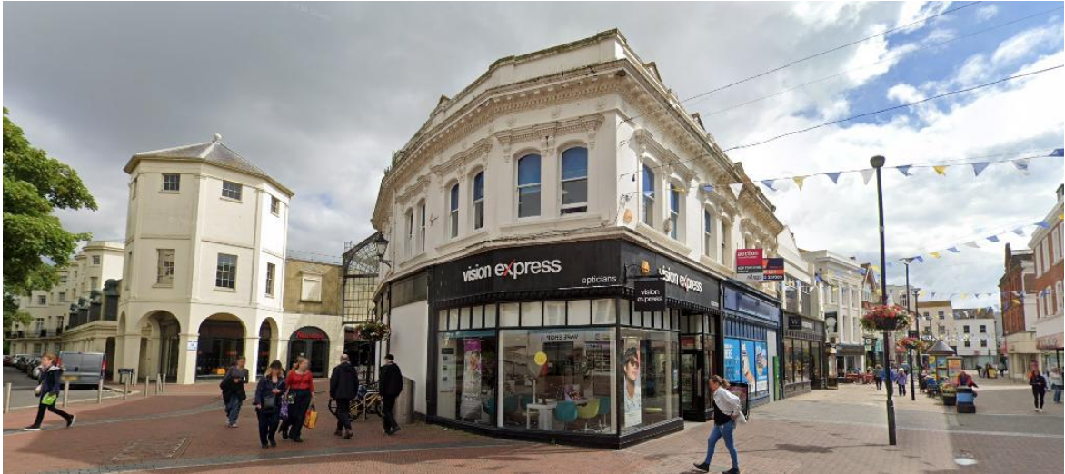
Above: The Site
