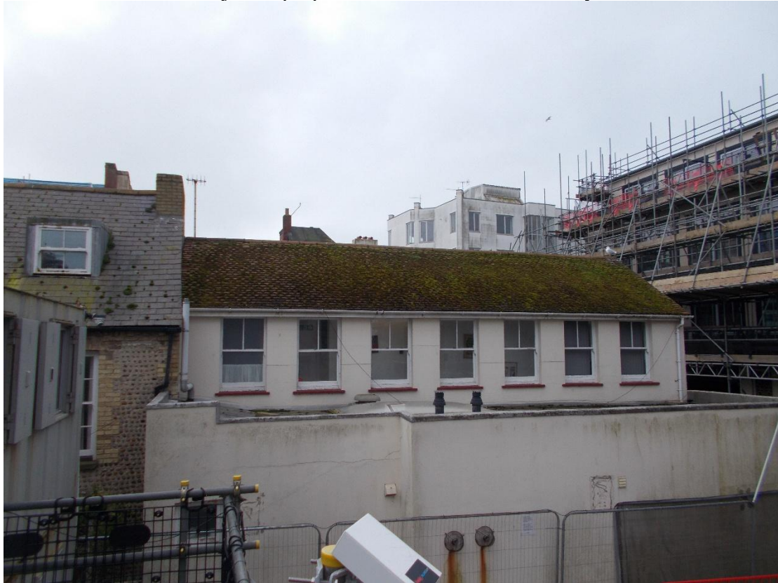
South adjacent properties – St Claires Community Hub
