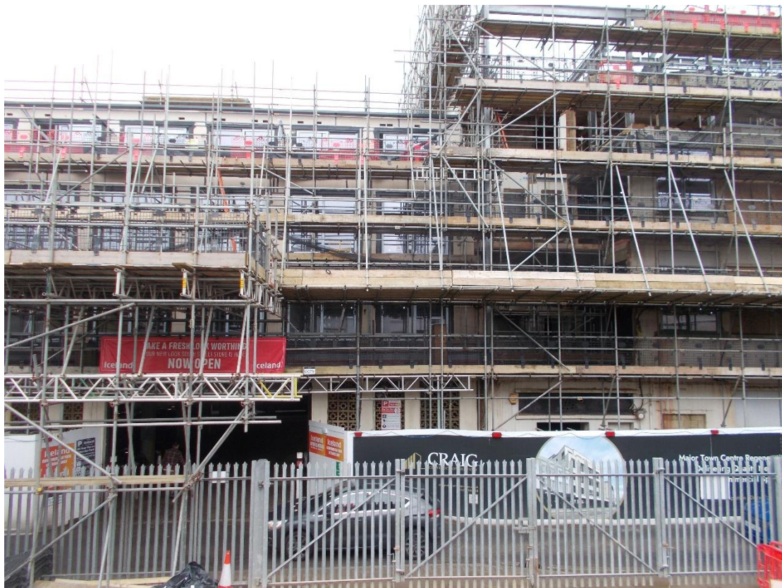
West adjacent property – under development residential flats
