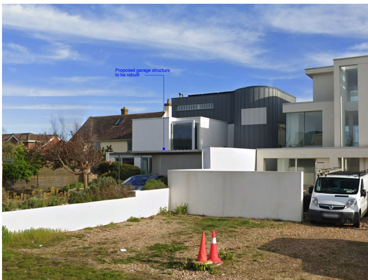
PHOTOGRAPH OF EXISTING FRONT ELEVATION (taken outside no. 98)
