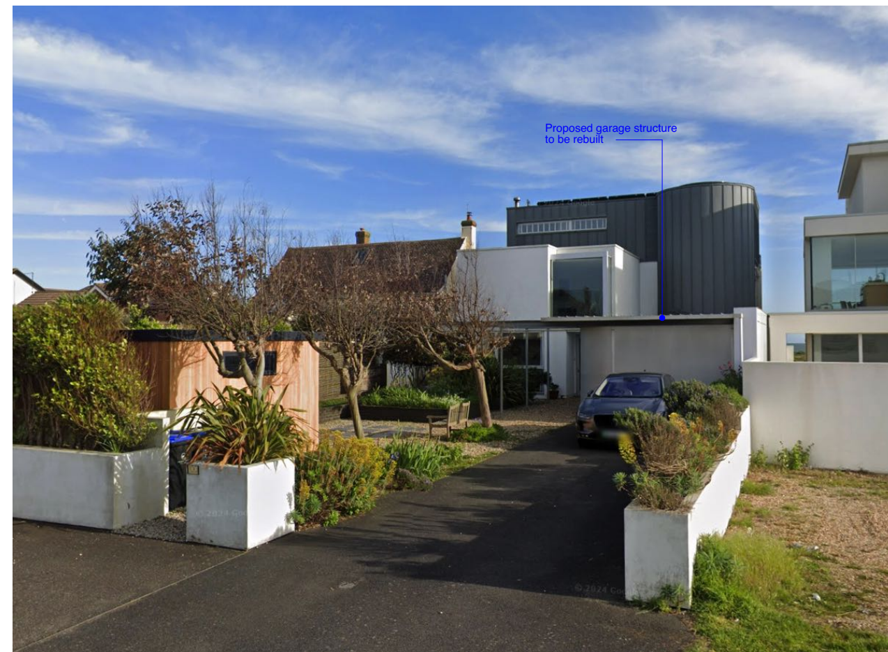
PHOTOGRAPH OF EXISTING FRONT ELEVATION
