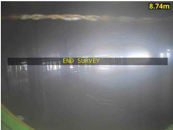
1_S18_Upstream_Line 2.jpg, 00:00:32, 8.74 m Finish node, other special chamber, reference: Line 2, OPEN IN BASEMENT
