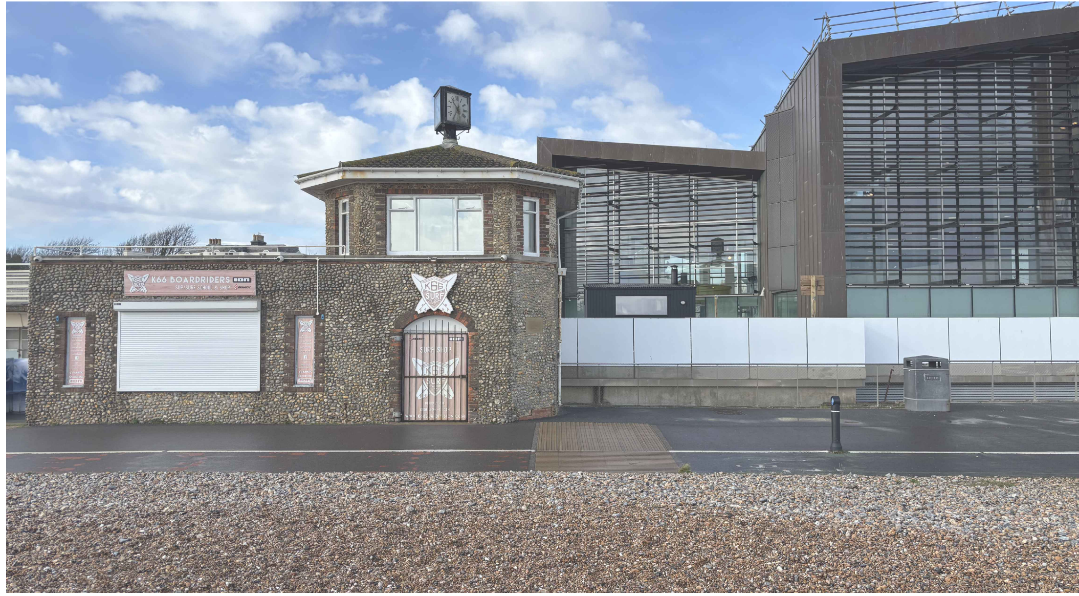
Site Photo - South Elevation
