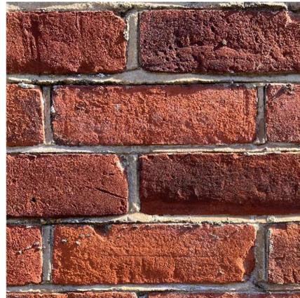
Obliquely illuminated Edwardian brickwork showing undulations and surface texture.
