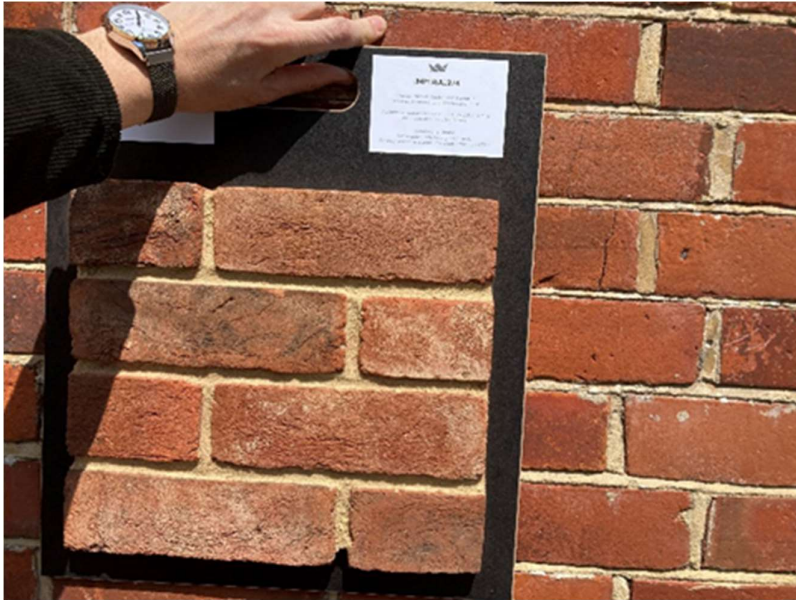
Imperial Bricks Reclamation Weathered Soft Red (Handmade): View of sample board held against existing brickwork
