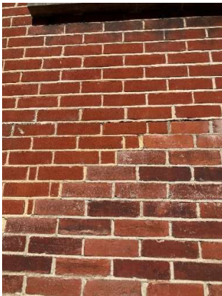
Area of brickwork repair to New Road stair showing highlighting tonal variation in original Edwardian brickwork (lower portion).
