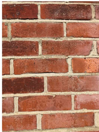
Typical area of original Edwardian brickwork.
