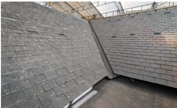
SSQ Del Carmen (quarried North-West Spain)
