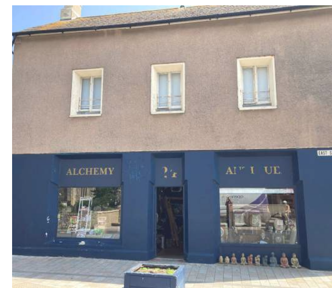
Fig. 15: Close-up view of East Street Building showing existing pebbledash
