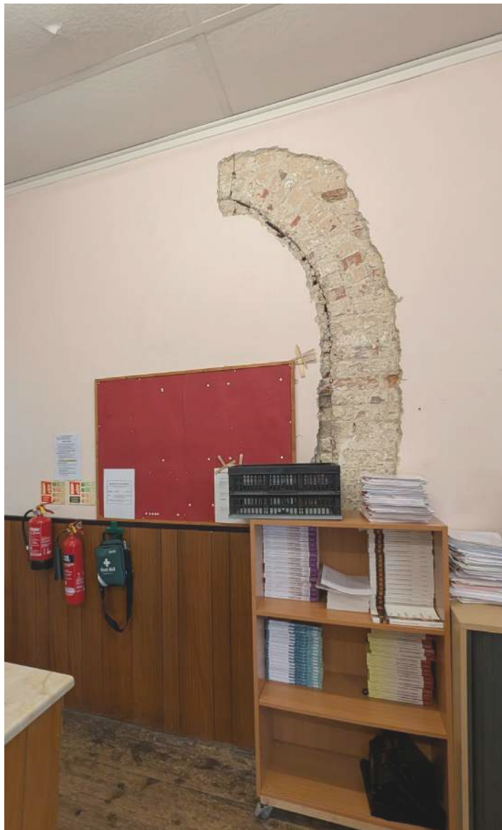
Fig. 48: Existing photo of original brick arch reveals discovered
