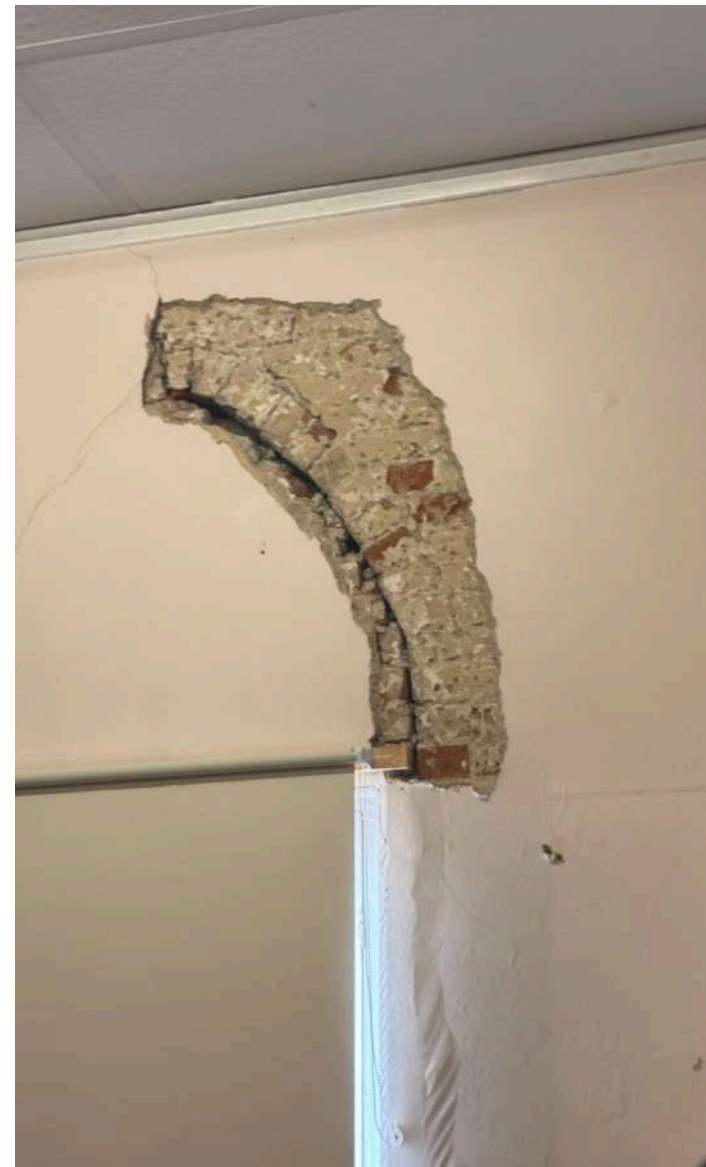
Fig. 49: Existing photo of original brick arch reveals discovered
