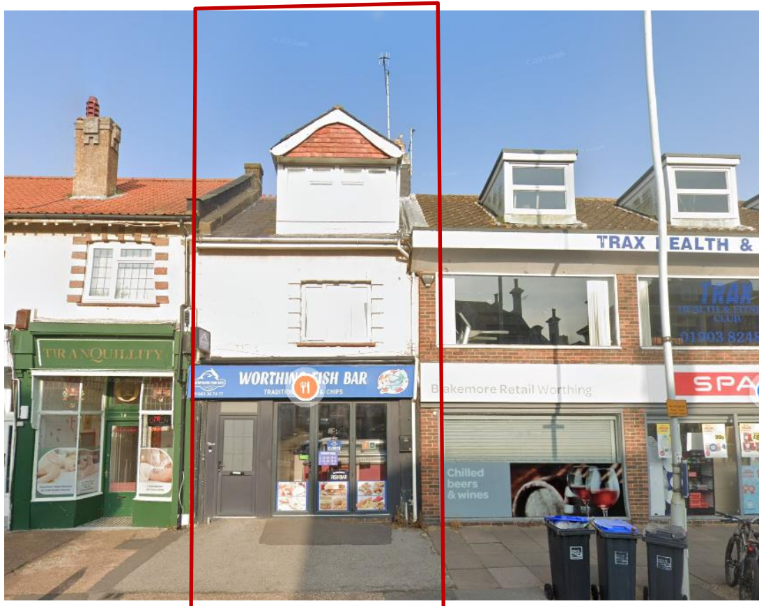
PICTURE OF THE 74 HEENE ROAD PROPERTY
