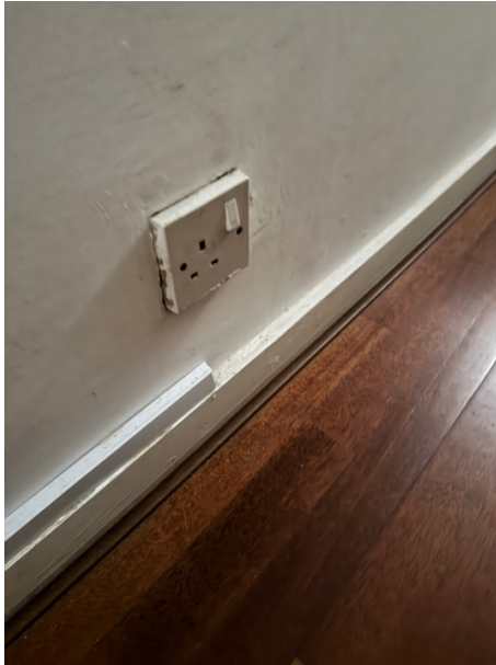
Existing non-original skirtings
