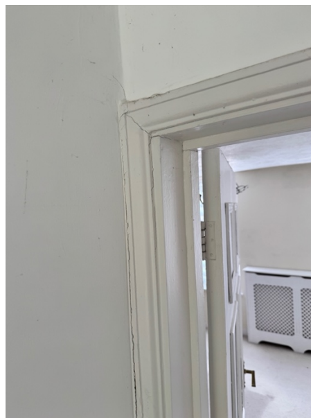
Existing non-original architrave to front bedroom
