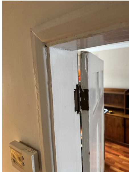
Existing non-original architraves
