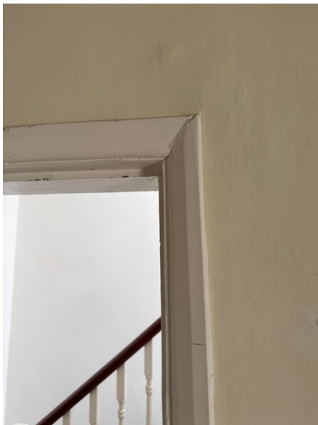
Existing non-original architrave to rear bedroom
