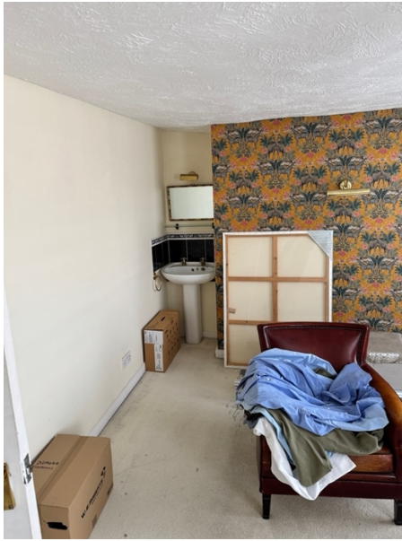
Chimney blocked up, modern basin in room and plain skirtings.
