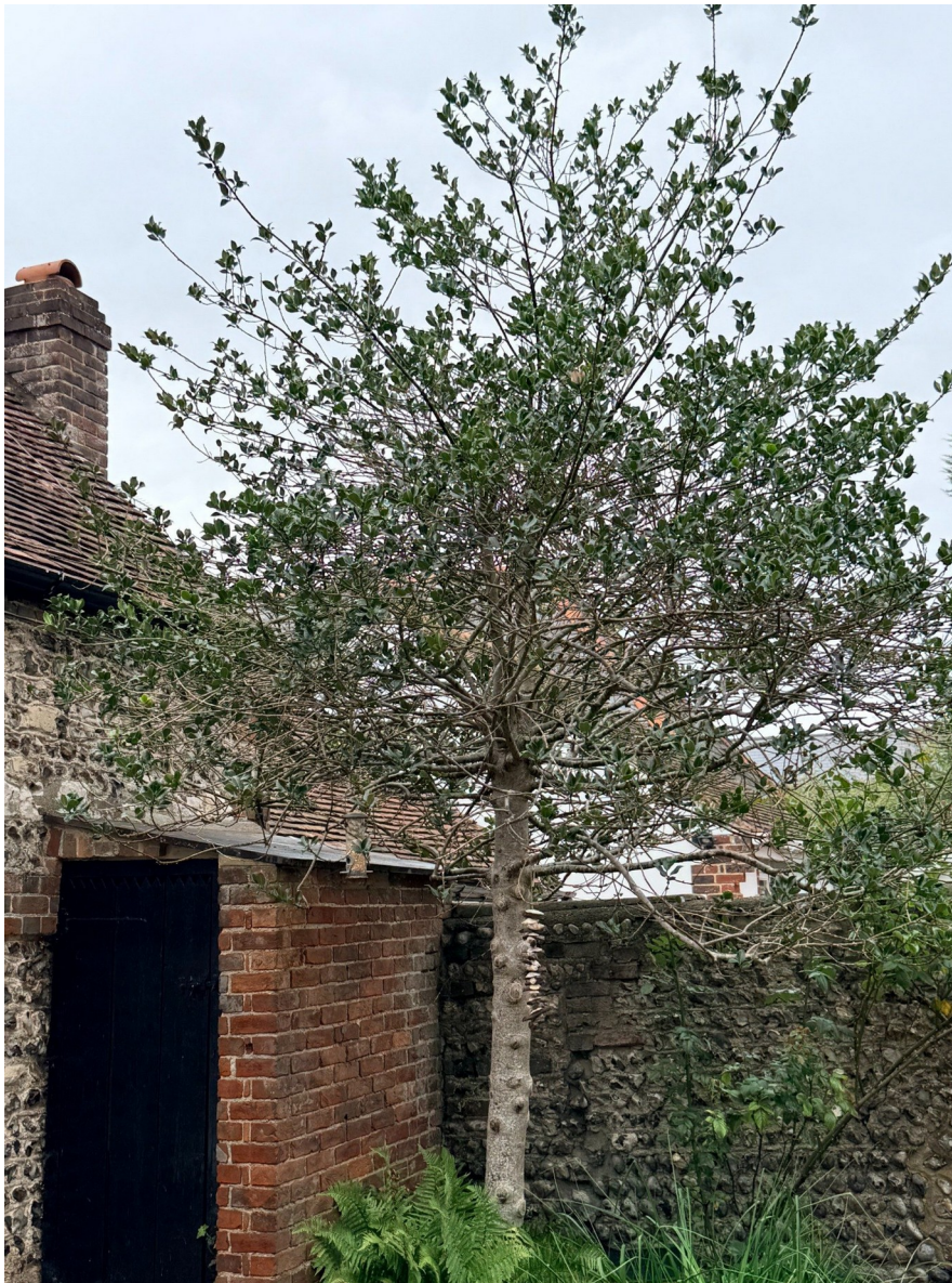
Photograph T6-A. Overall view showing the Holly immediately adjacent to the roof of the main house.
