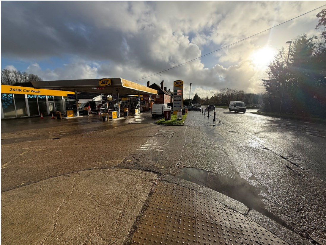
Photo 4: The forecourt is constructed of concrete slab.
