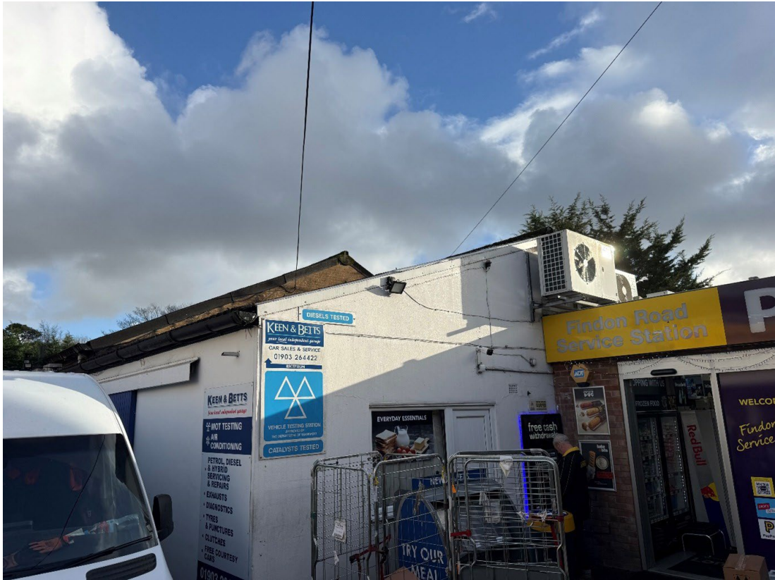
Photo 6: The workshop located on the Site.
