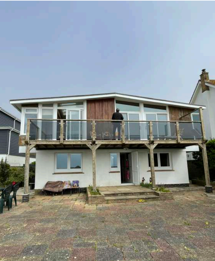
8. South elevation from rear garden
