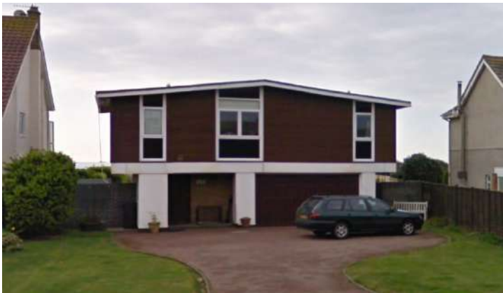
154 Old Fort Road in 2009 showing original timber cladding
