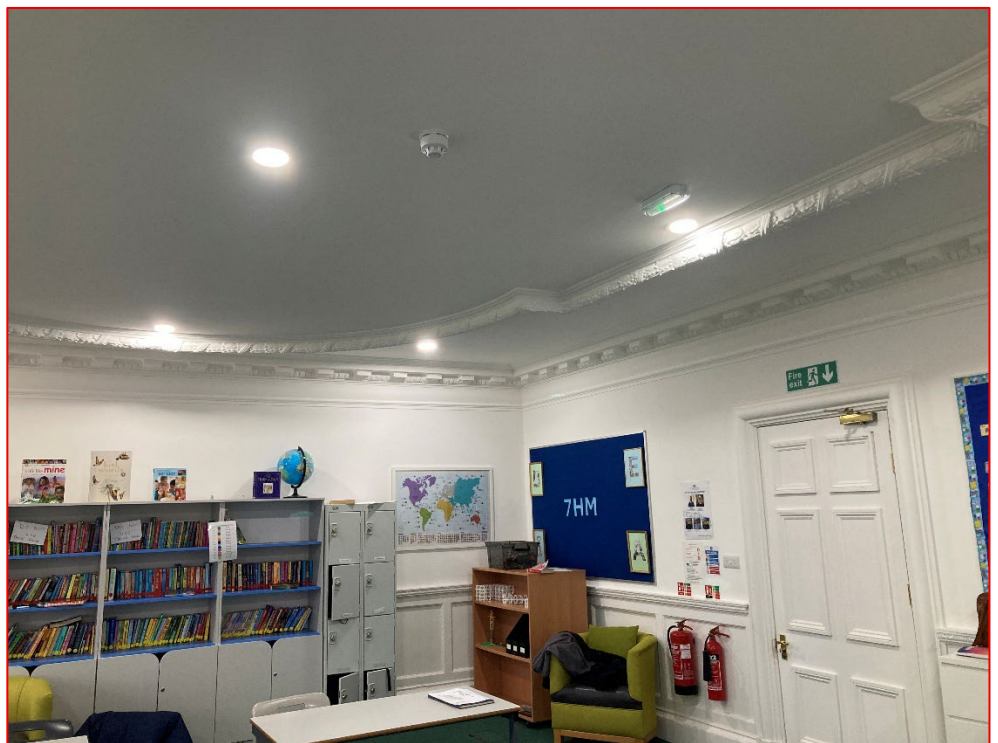
Plate 9 Room 19 (First Floor) following its renovation as part of the conversion of the building into a school illustrating the high standard of decorative finish that is evident throughout the building.
