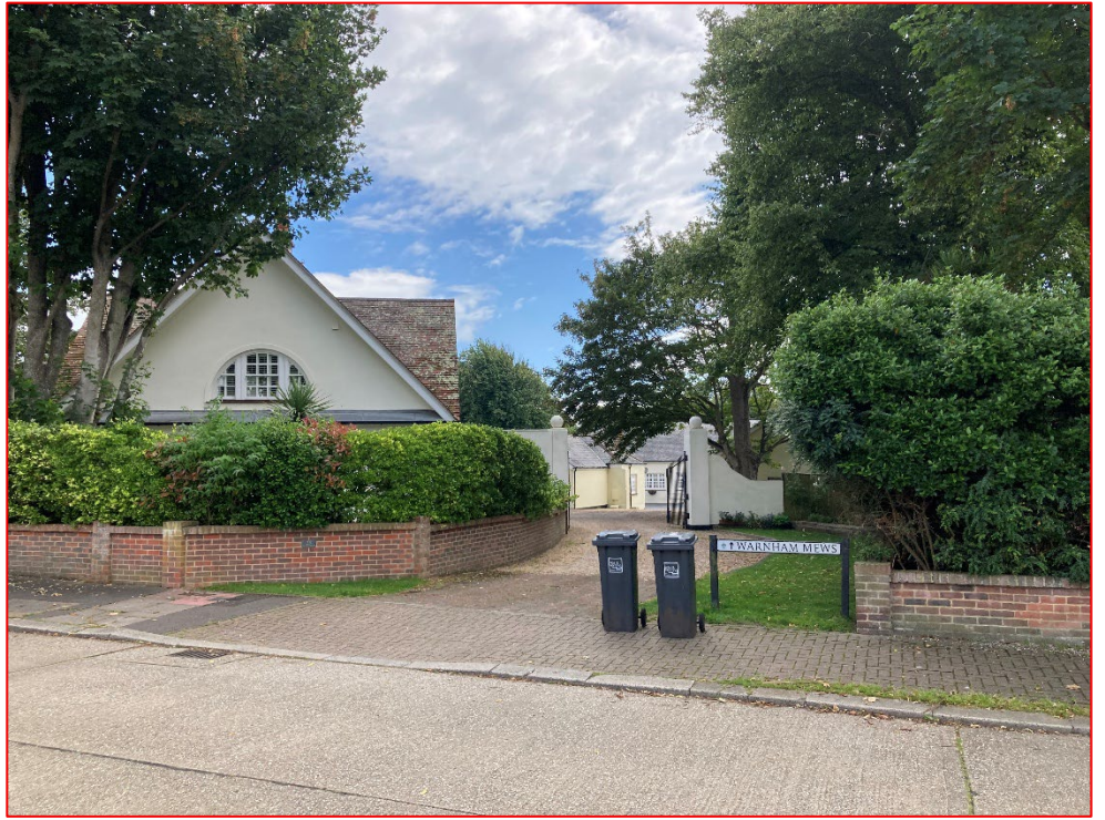
Plate 8 Summer view of the circa 1999 'Gatehouse' (left), which fronts Warnham Road to the west of the site.
