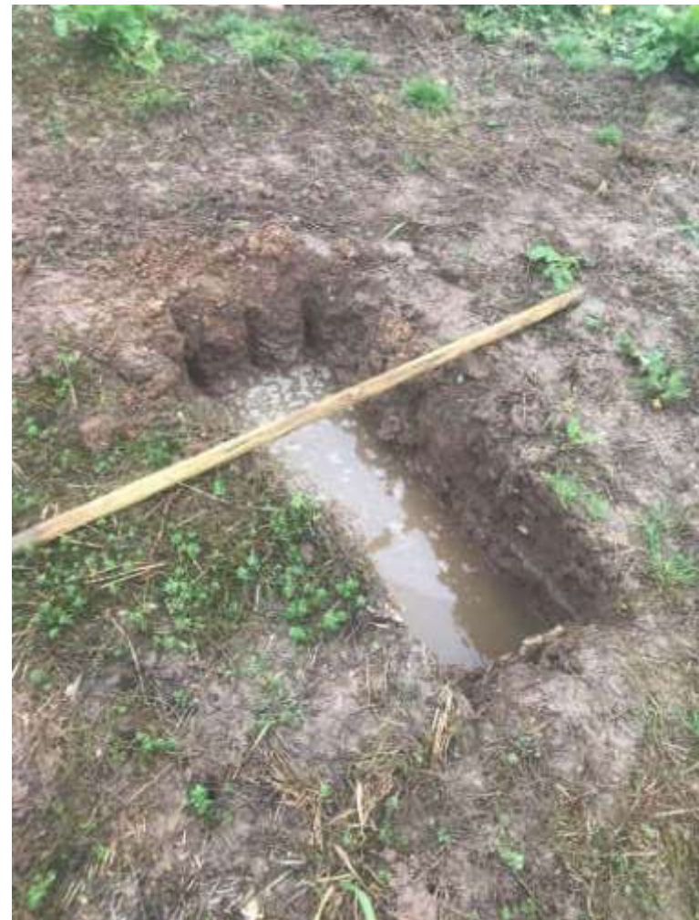
Plate 8: TP4 during soakage testing
