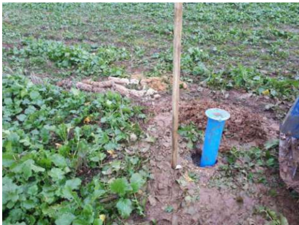
Plate 2: WS5 with well cover (before addition of cement)
