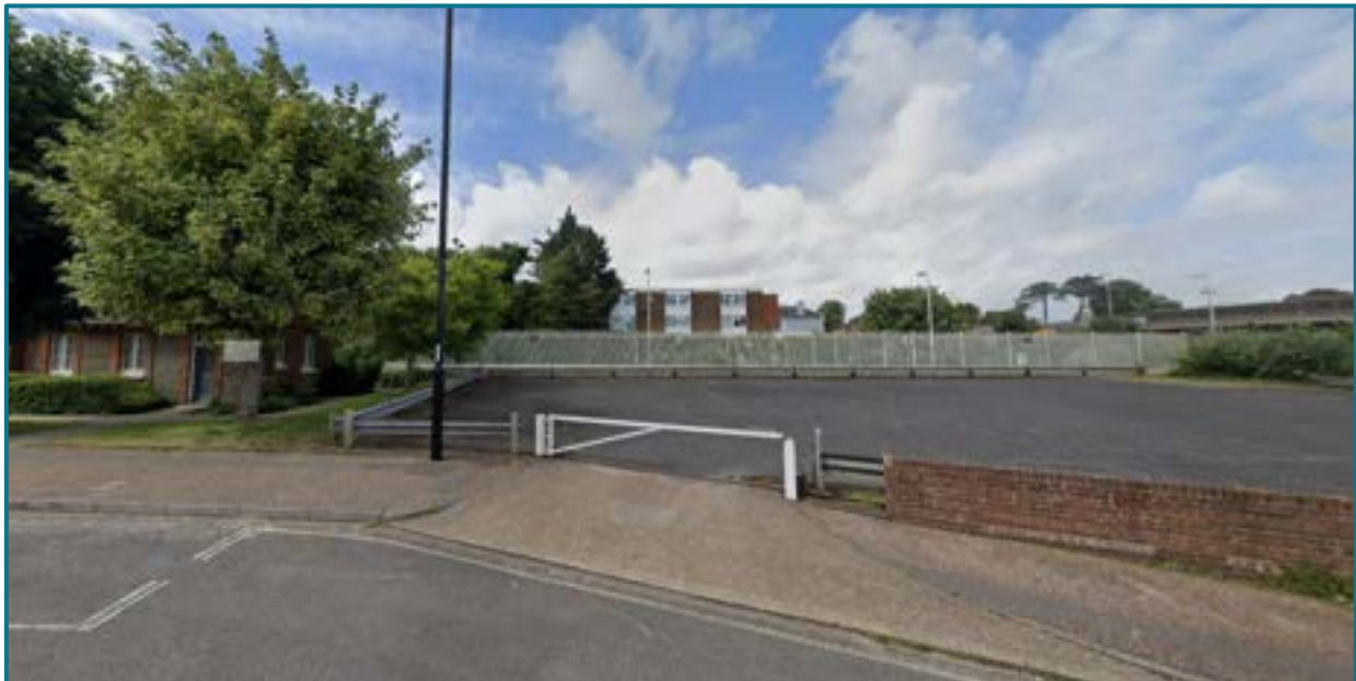
Figure 5.1 – Existing Access to the site
