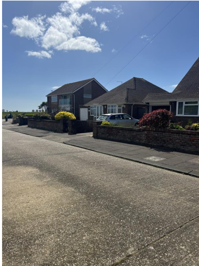
Image 6: Streetscene looking along St John's Avenue from a different angle, showing (left) the two-storey flats, (centre) a single-storey bungalow, and (to the right of centre) a taller chalet bungalow with a visibly higher roof ridge. The image demonstrates in a single frame both the two-storey context opposite the site and the height variation that already exists between properties on St John's Avenue. The open grass and seafront are visible to the left.
