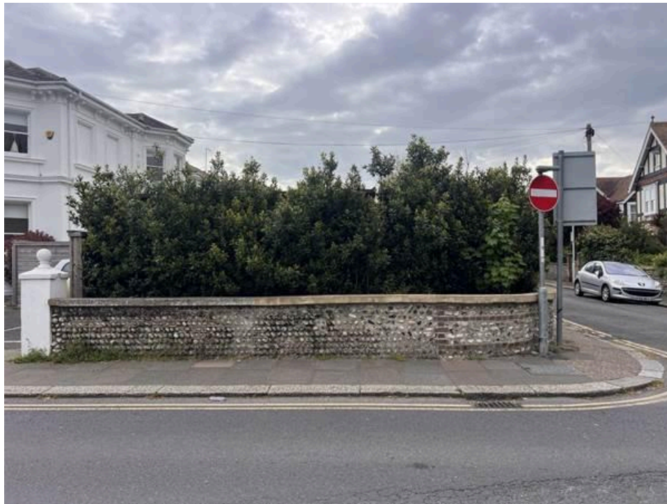
Figure 5. Long elevation along Crescent Road, showing the continuous evergreen screening above the boundary wall along the western edge of the site.
