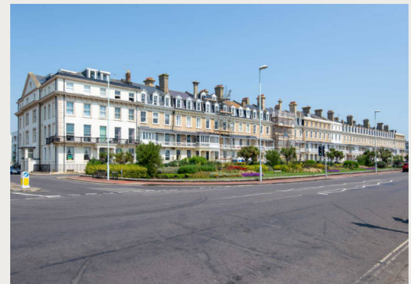
Figure 2: Contemporary image of Heene Terrace showing the missing canopy to the western bookend.
