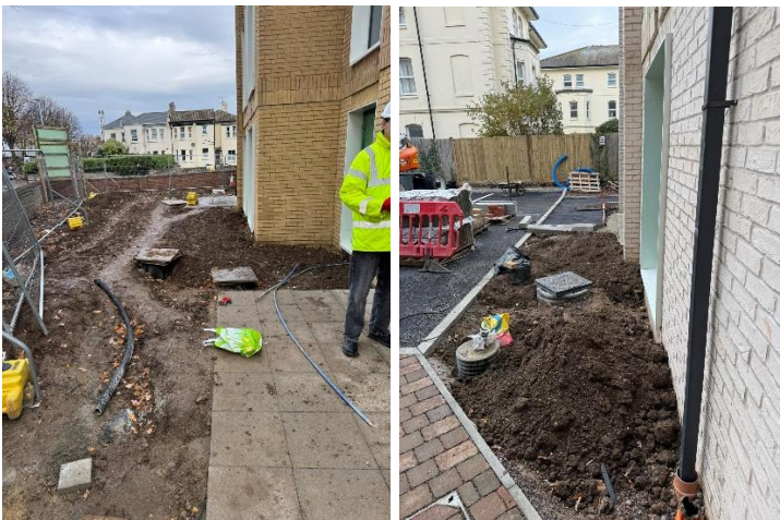
Inspection chambers in place, covers to be set to finished topsoil level.
