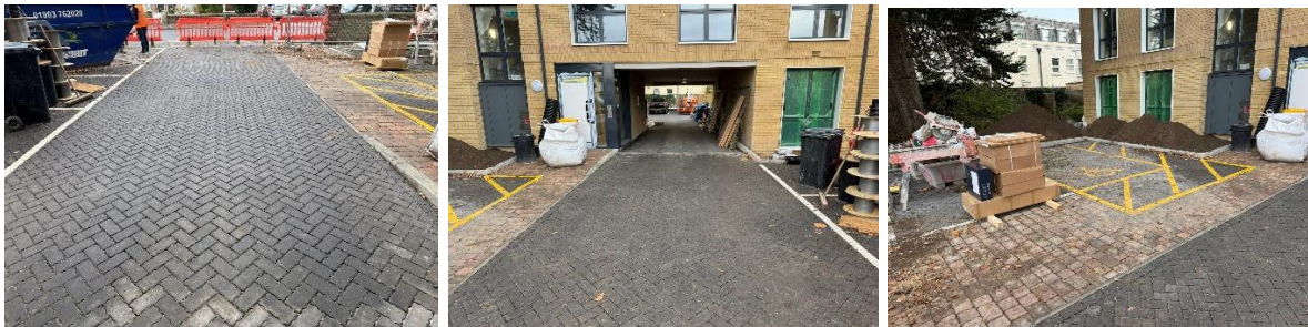
Permeable paving to entrance and parking area.
