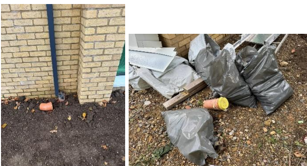
Rainwater downpipe awaiting final connection and rodding eye ready for cover once topsoil placed.
