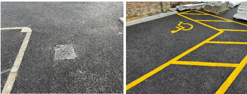
Permeable tarmac to rear car park.
