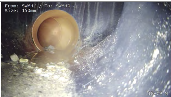
Junction at 9 o'clock, diameter 100mm
