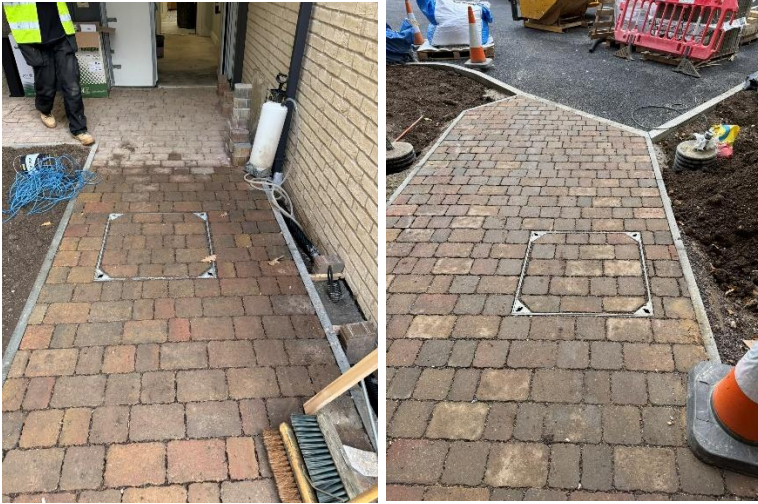
Permeable paving to footway with gritstone brushed in.
