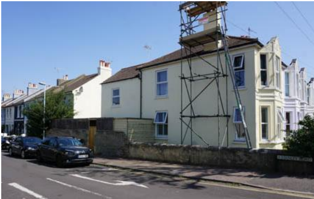
Figure 2 – Stanley Road side elevation of the property
