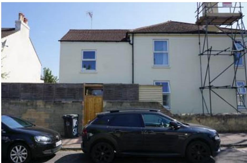
Figure 3 – West side elevation showing boundary fence and timber outbuildings
