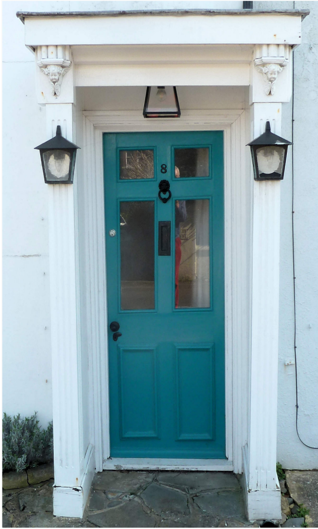
Existing Porch Surround of 8 Warwick Place
