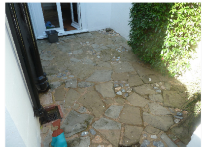
Existing Paving in Yard
