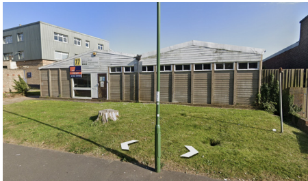
Figure 3: North-west view documenting the existing street-facing elevations as viewed from Marlborough Road. These figures illustrate the current dilapidated state of the single-storey structure and the aging, sub-standard industrial stock the proposal seeks to replace
