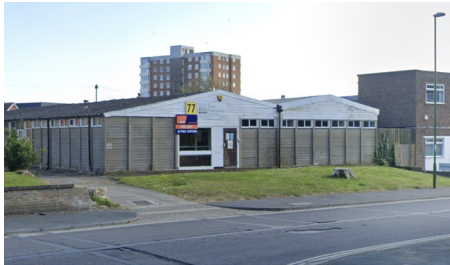
Figure 2: North-east view of site from Marlborough Road
