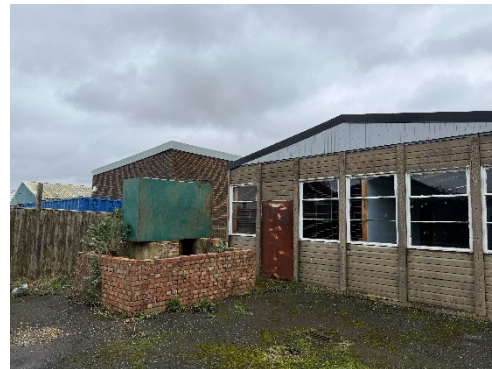
View facing the rear of B1
