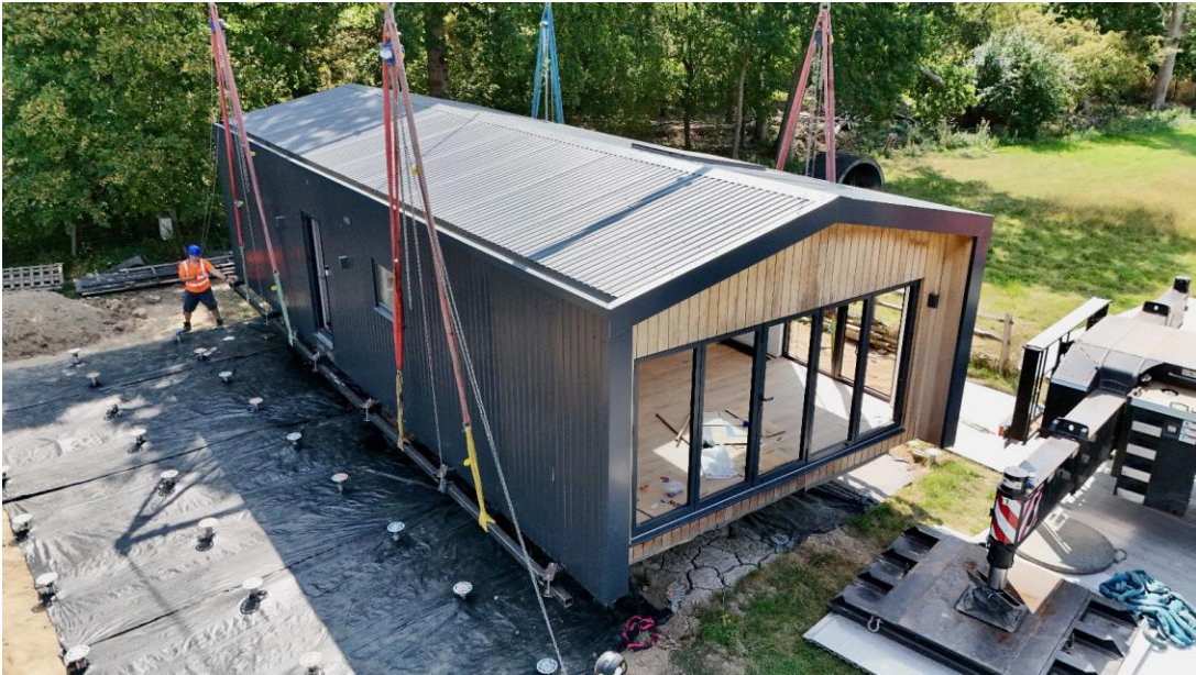
Figure 2 – Mobility of Caravan by Crane
