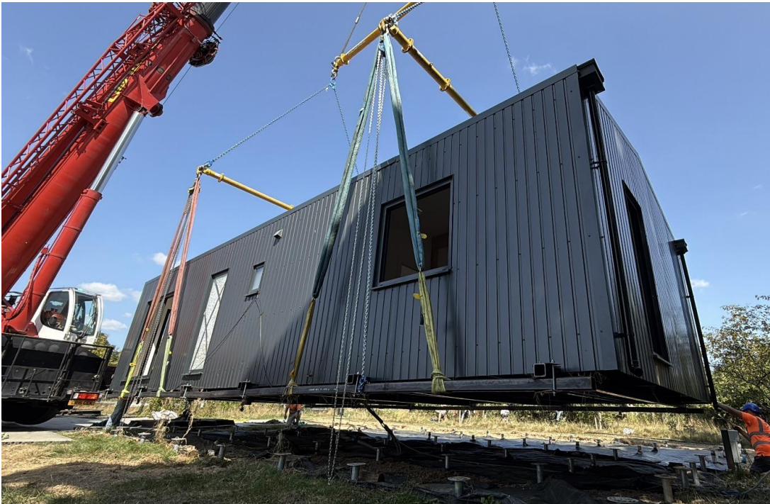
Figure 1 – Mobility of Caravan by Crane
