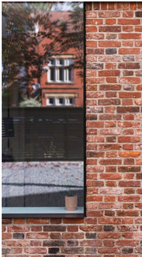
Dark framed windows / Facing Brick
