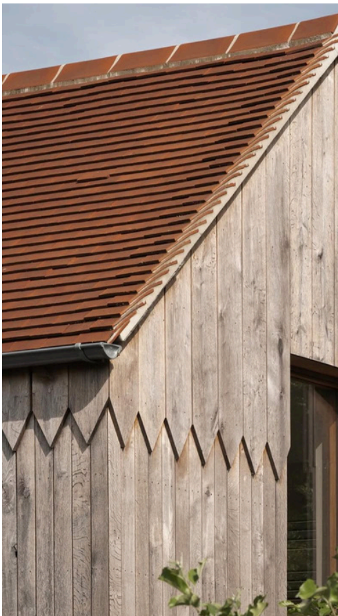
Red/Brown Roof Tiles
