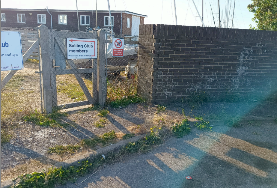
PRECEDENCE Access Gate from the car park serving the Sailing Club on the North/West Elevation
