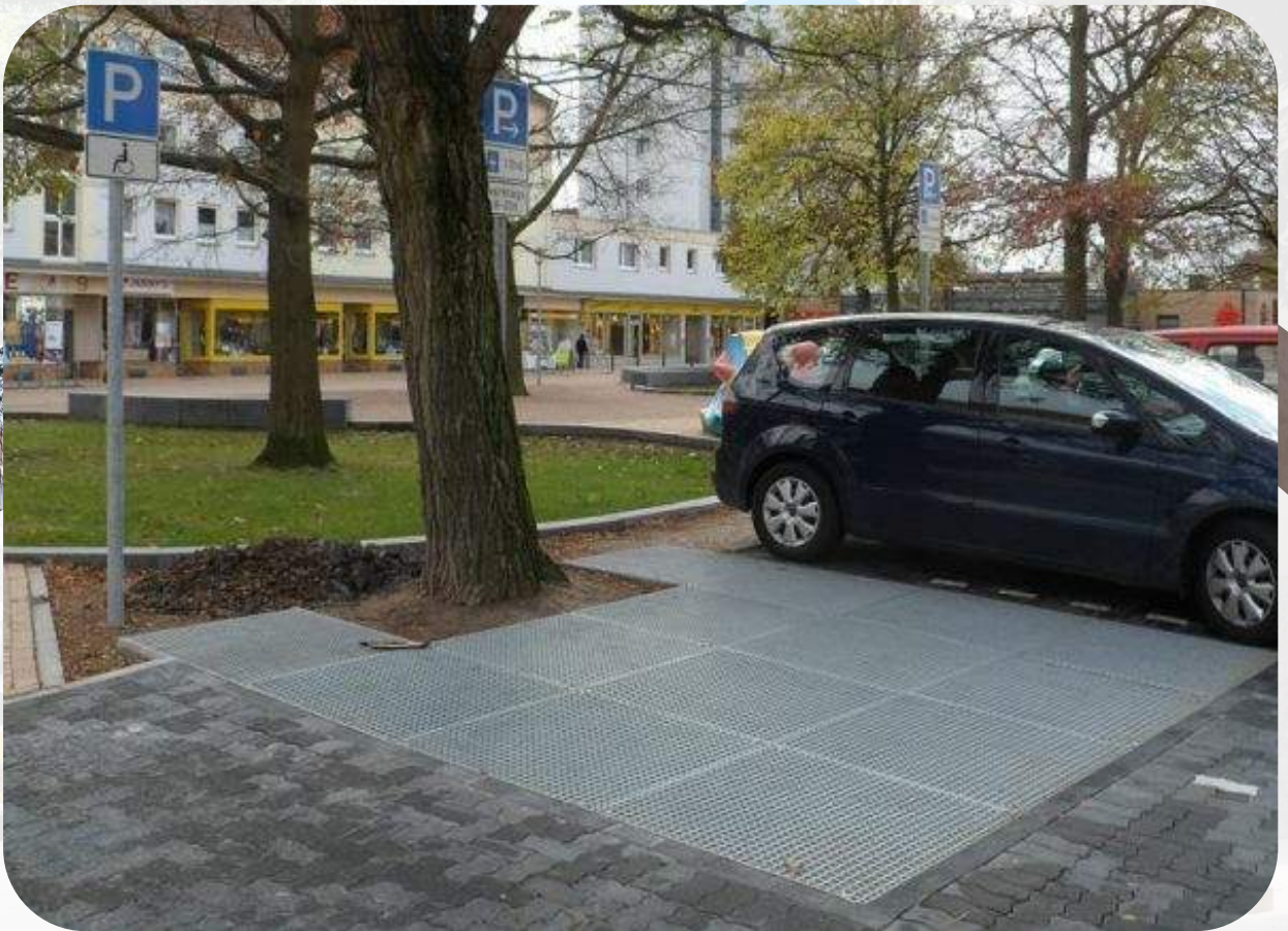
Light duty install in a carpark, heels-safe mesh finish.
