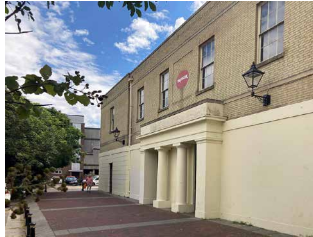
3.13 The north facade
