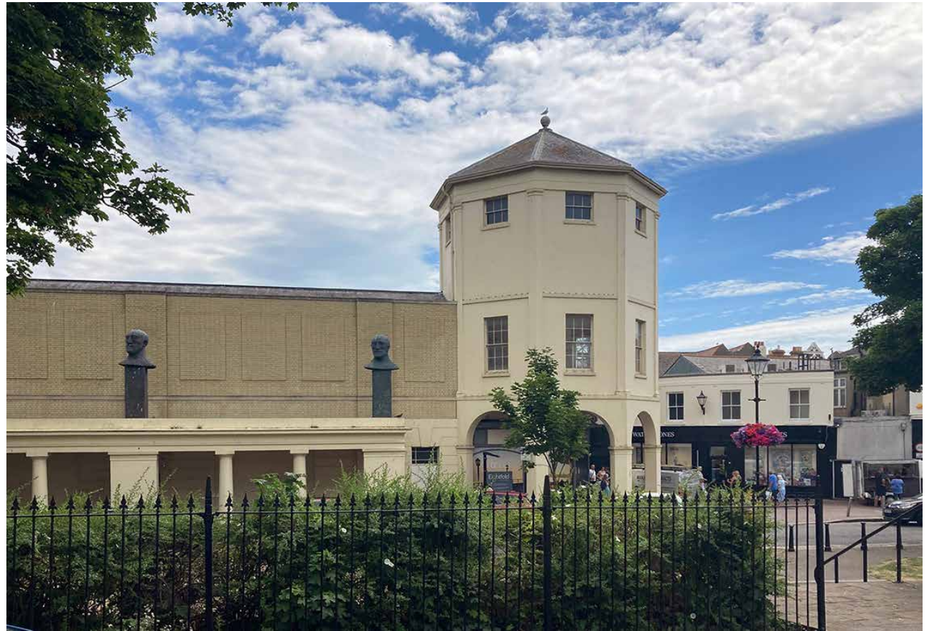
3.19 View of the two heads at the south end of the Desert Quartet, seen from the west, in Liverpool Terrace
