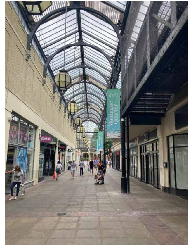
3.16 In the arcade looking north
