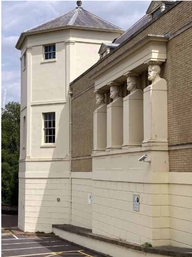
3.12 The north octagonal tower and the entablature with Atlas columns
