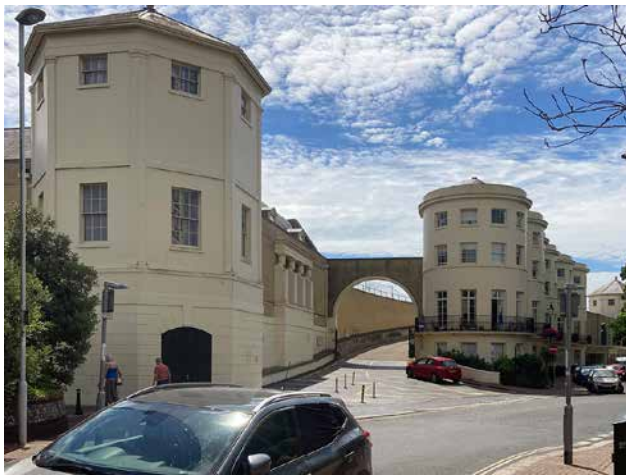
3.11 The vehicular access to the roof of the Montague Quarter
