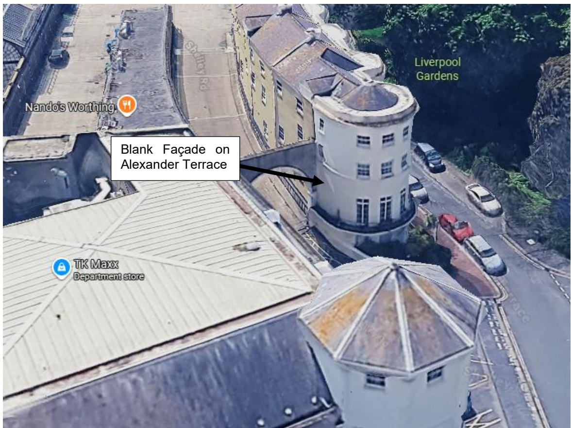
Figure 3 - Blank Facade on Alexander Terrace
