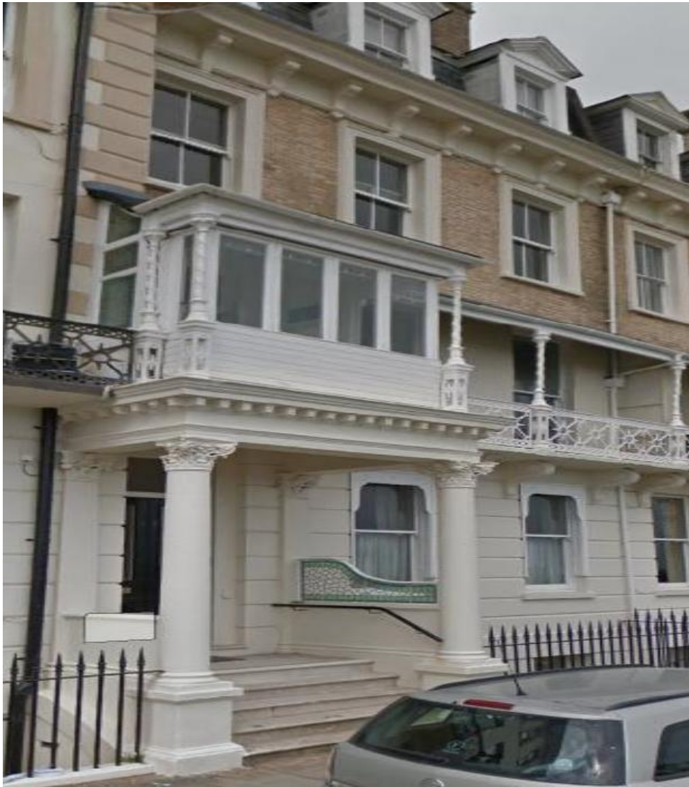
Figure 9: View of the subject property prior to scaffolding works
