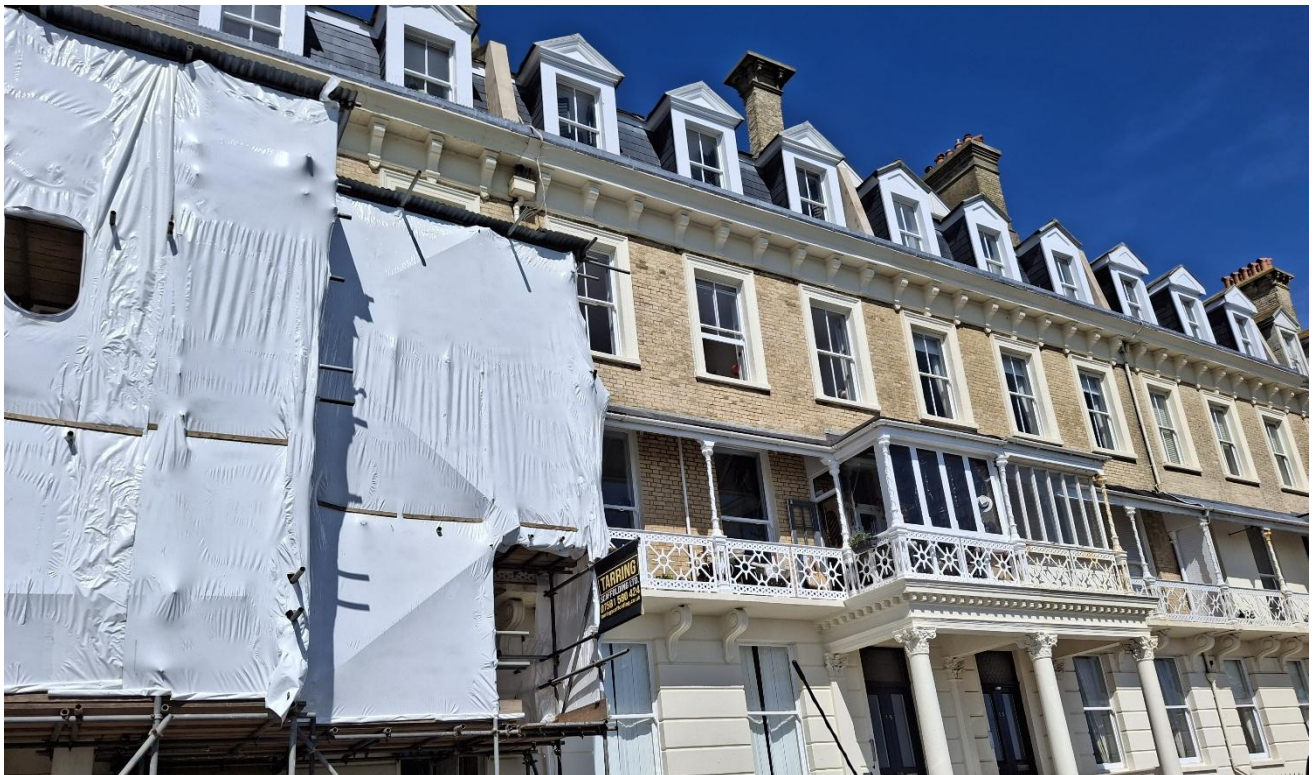
Figure 7: Close up view of Heene Terrace and Subject property (to the left) currently obscured by scaffolding
