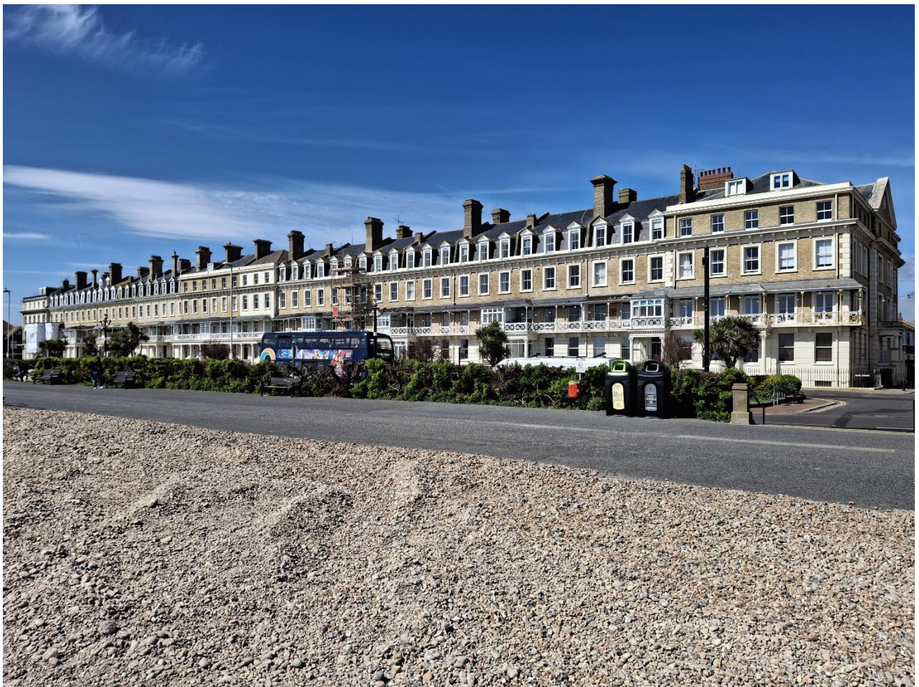
Figure 6: Complete view of Heene Terrace
