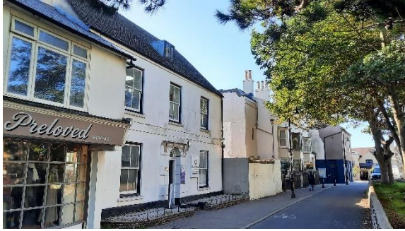
View of the street frontage, looking southwards down East Street; the site is just visible at the far end
