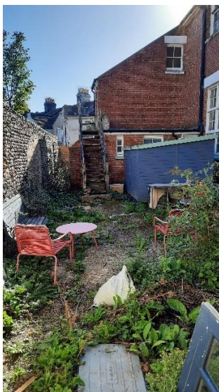
Rear of the building, looking east
