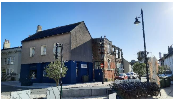
General view of the site showing its prominent position at the intersection of East Street and New Road
