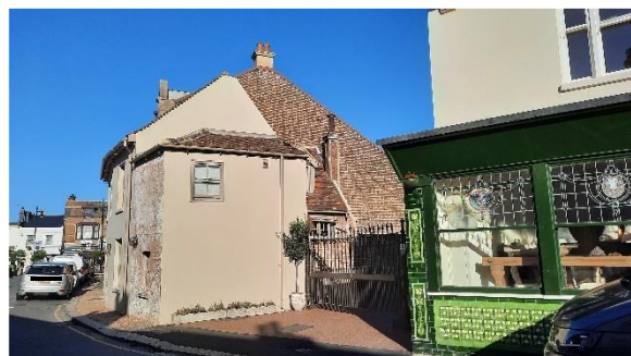
Looking west at the end elevation of the building visible upon turning the bend in New Road
