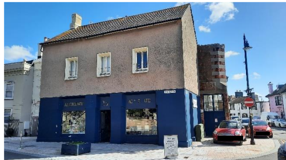
The west elevation of the old school building
