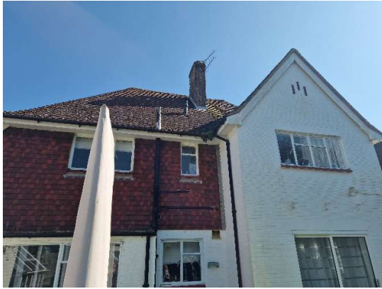
Figure 5: Tiles on the rear façade.
