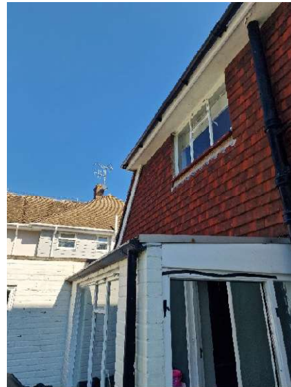
Figure 2: Western side of the residential dwelling.
