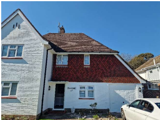
Figure 7: Front view of the residential
