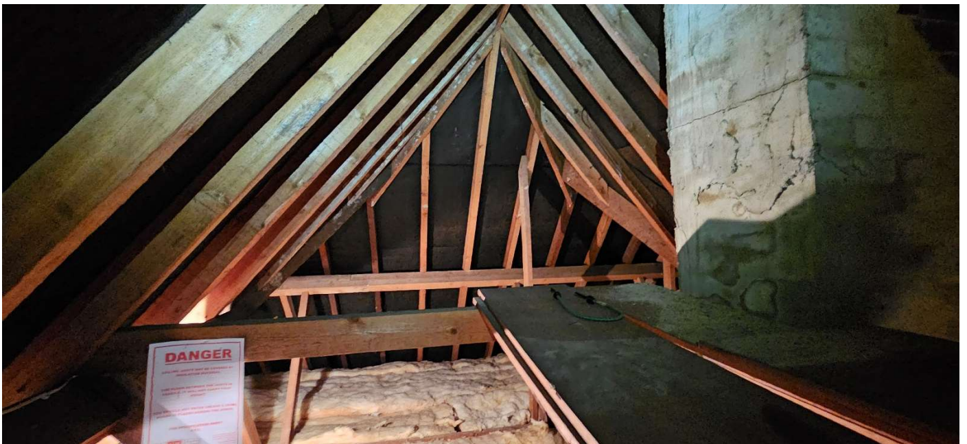
Photo 4 – Loft void from the hatch facing south
