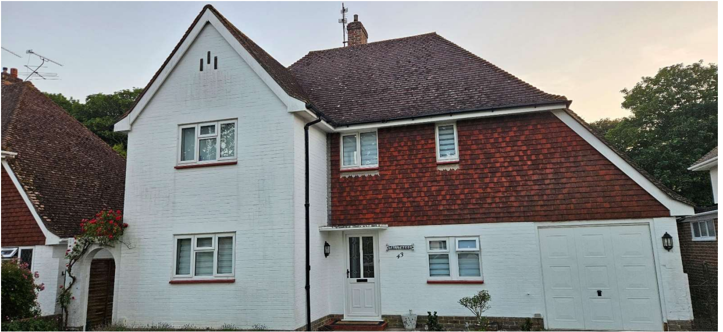
Photo 1 – Front of the property (east elevation)
