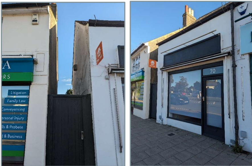
Above: Existing front elevation
