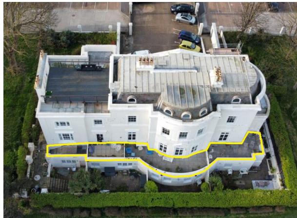
Figure 1: Areal image of rear terrace work area
